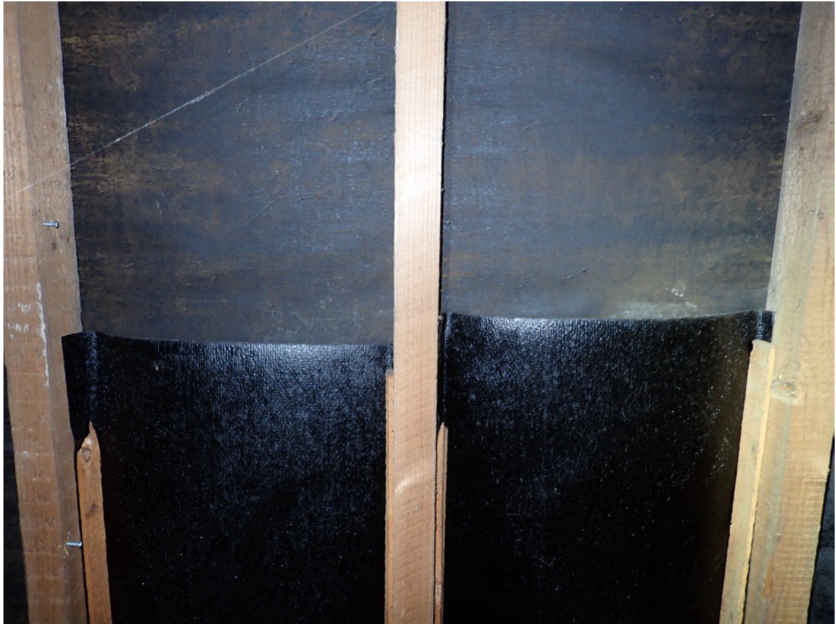
9 – The roof lining is. In reasonable condition with no gaps or tears.
