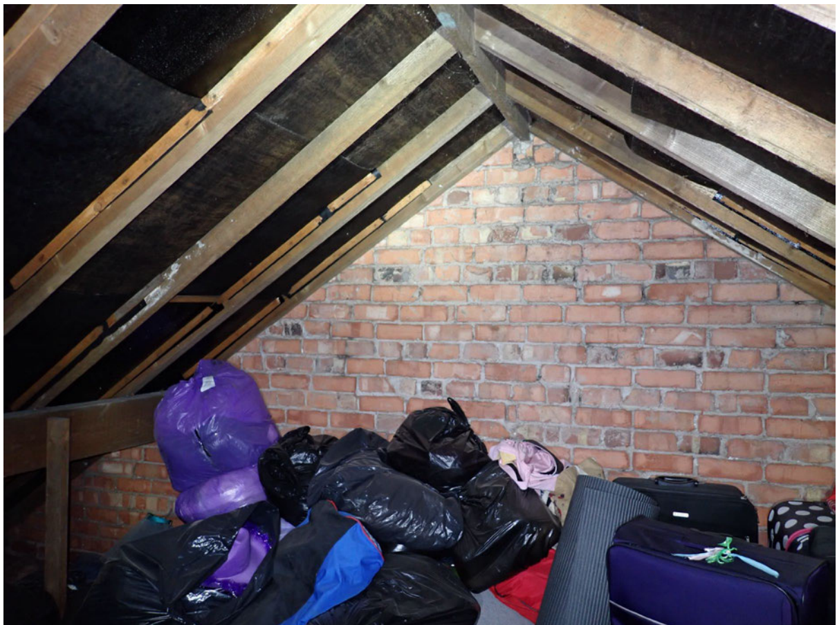
8 – The house has a single roof void which is lined with bitumen felt.
