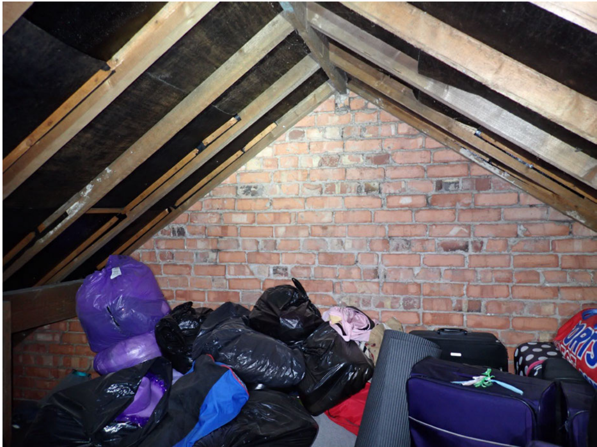
3.2a – The roof void.
