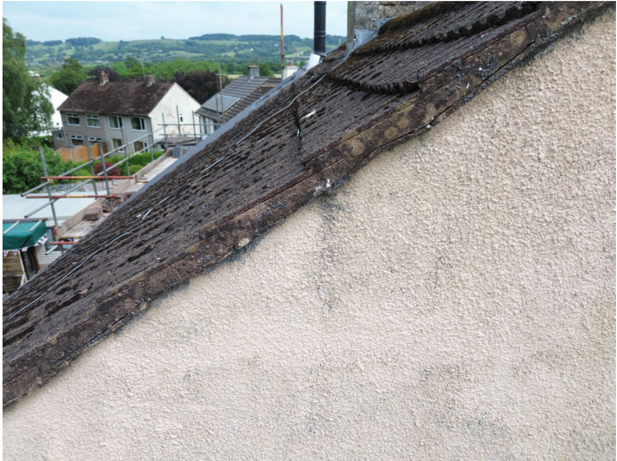
5 – End tiles at the verges are sealed with cement.
