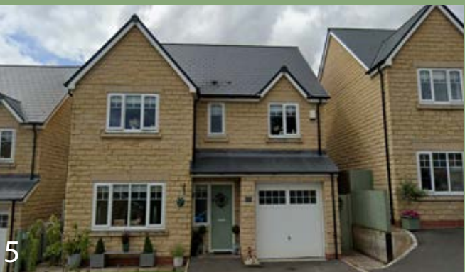
Detached, two-storey dwelling constructed in natural stone, reflecting a contemporary interpretation of traditional vernacular architecture. The front elevation is articulated through projecting gables creating a varied yet balanced composition
