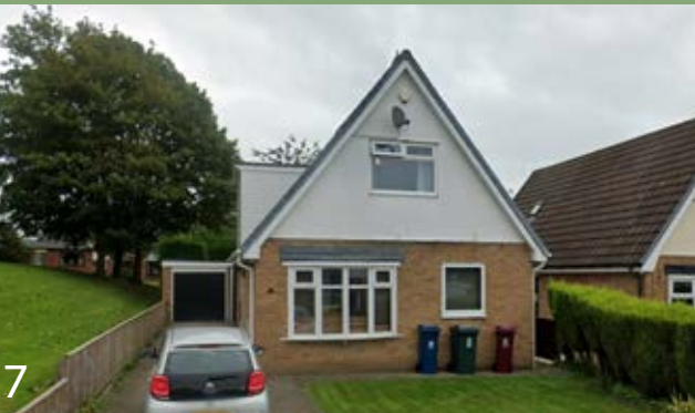
Detached dormer-style dwelling characterised by a prominent front-facing gable and a simple pitched roof form. The elevation combines facing brick at ground floor level with light render above, creating a clear horizontal division.
