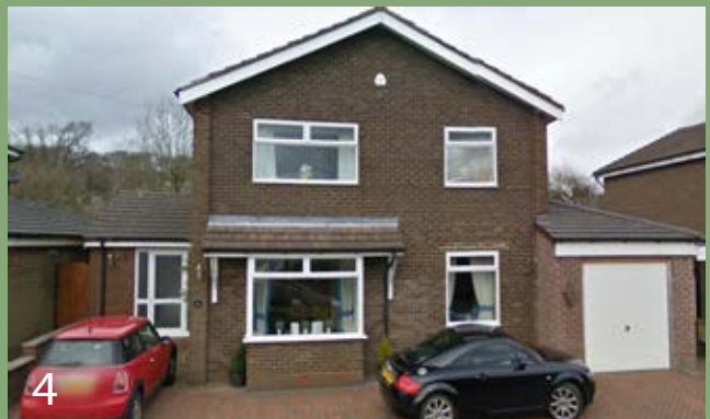
Detached, two-storey dwelling of simple, box-like form, constructed in brown brick with a shallow pitched roof. The front elevation is symmetrical in composition, with evenly spaced window openings and a central ground-floor emphasis created by a modest canopy projection.
