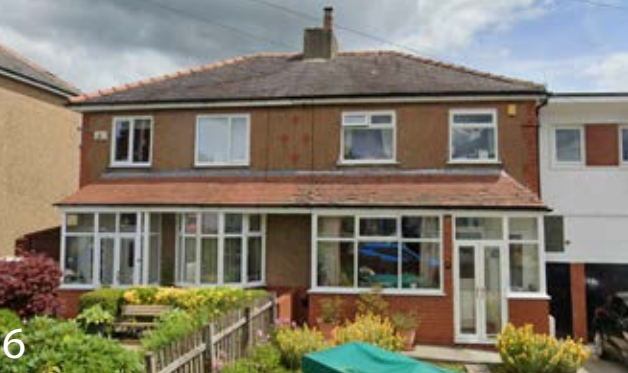
Semi-detached, two-storey dwellings constructed in brick and roughcast render. The front elevations are characterised by a continuous canopy and large ground-floor window openings, including bay elements.
