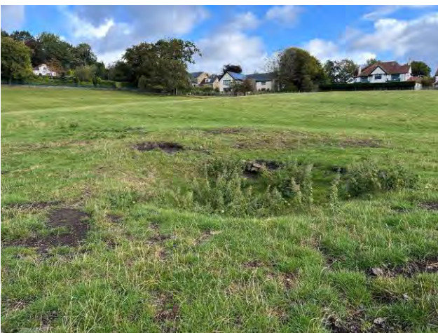
Figure 7 Circular depression on site, potential mine entry.
