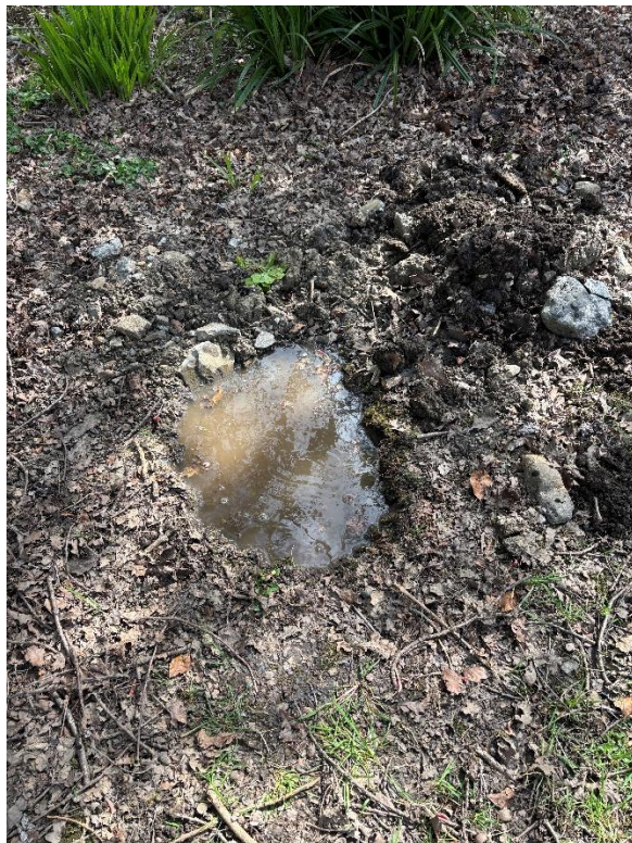
Image 2. Trial hole, backfilled with standing groundwater.
