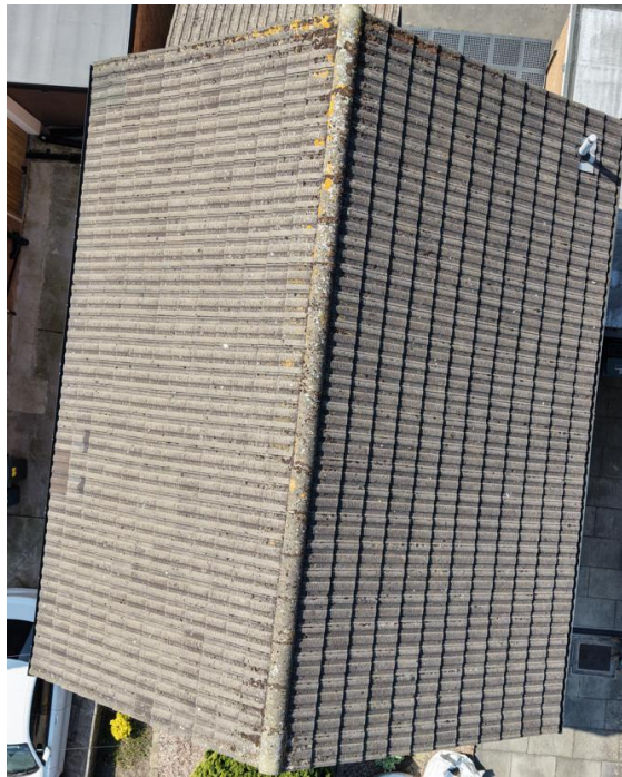
Photo 4. Overhead photo of roof.
