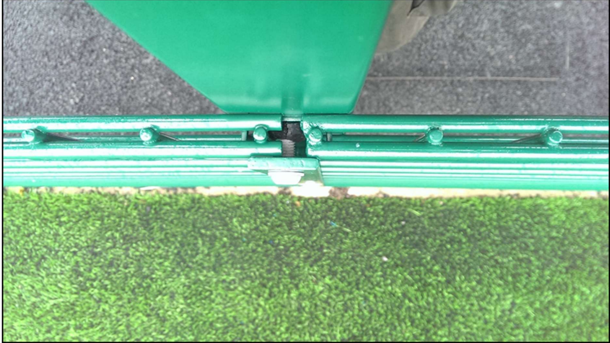
Figure 9: Image showing neoprene isolators
