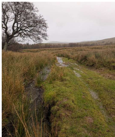
Fig 4 Drain/stream alongside track after culvert
