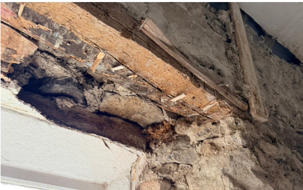
Image 5 Existing timber lintels
