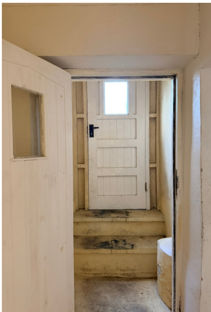
Image 9 Existing rear entrance
