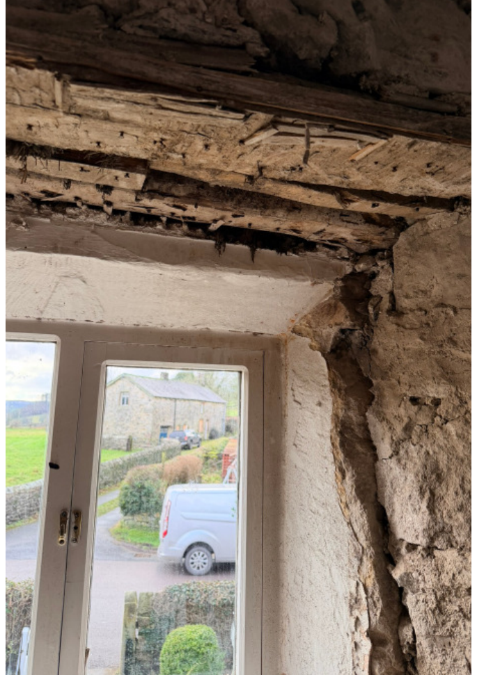
Image 5 Existing timber lintels
