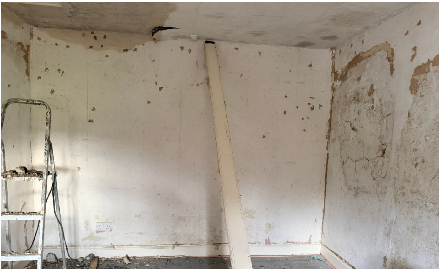
Image 7 Existing internal walls (landing)
