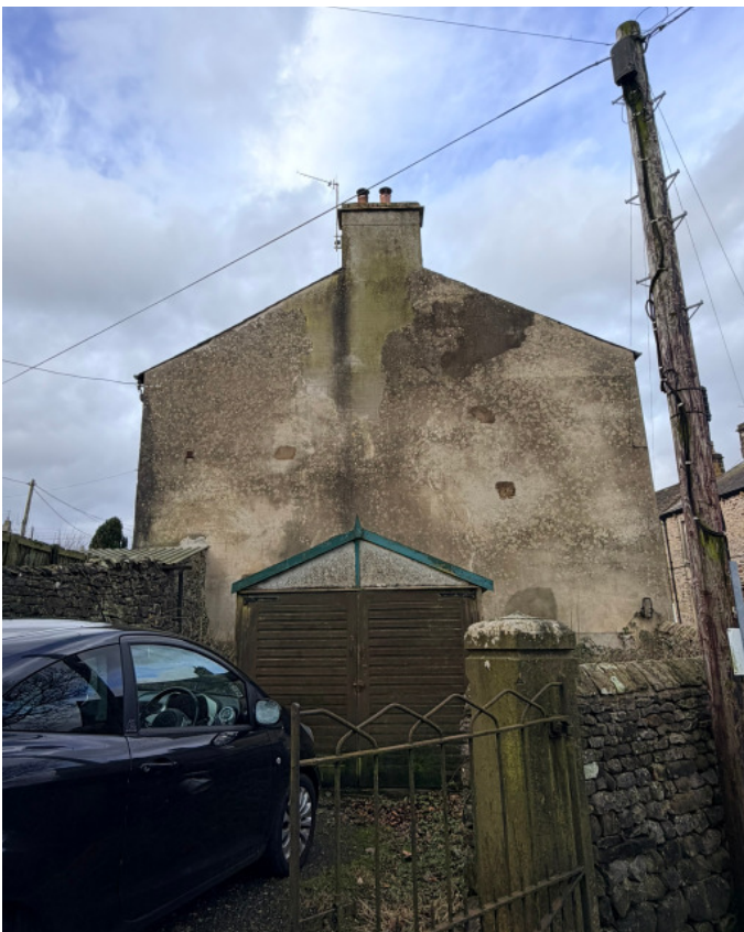
Image 2 Gable End - Sand / Cement Render
