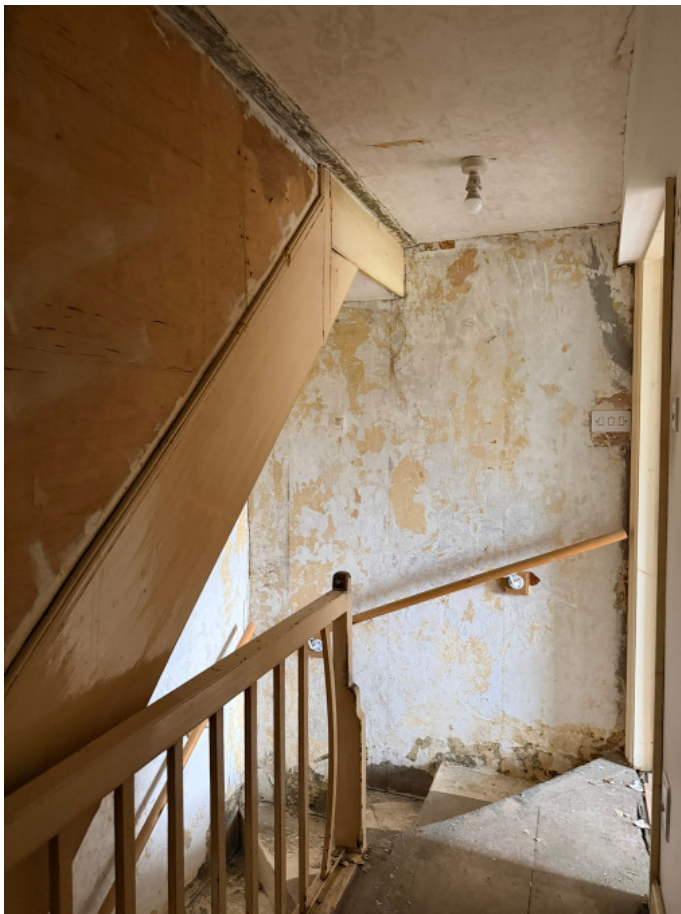
Image 7 Existing internal walls (landing)
