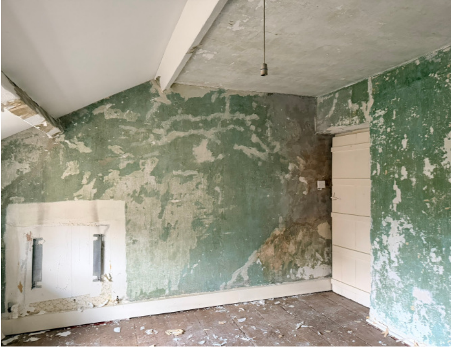
Image 6 Existing internal walls (bedroom)
