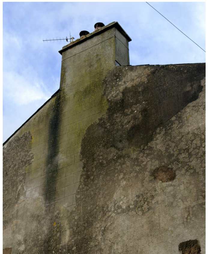
Image 3 Gable End - Sand / Cement Render
