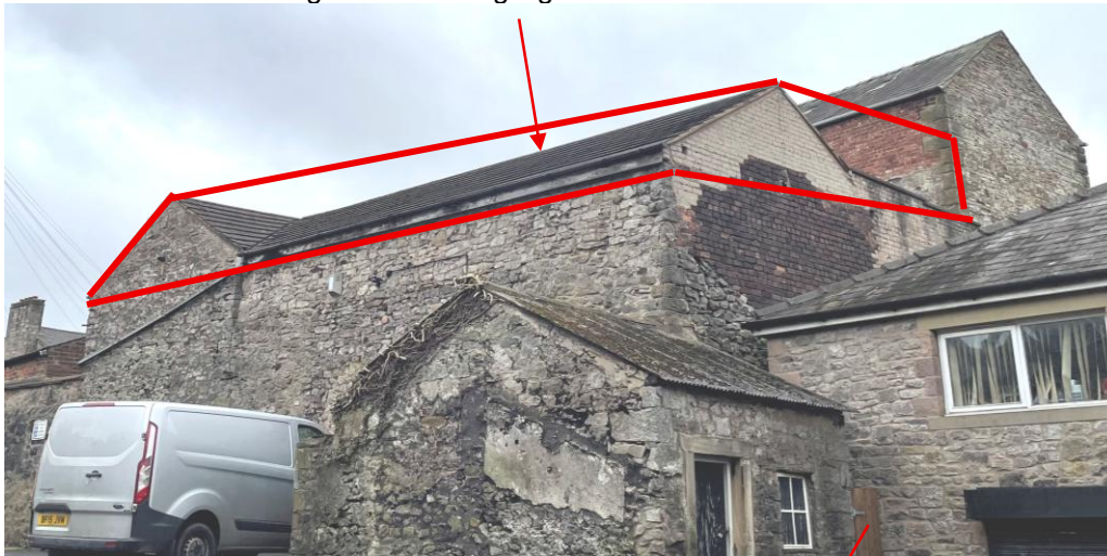
Rear northeast Elevation.
