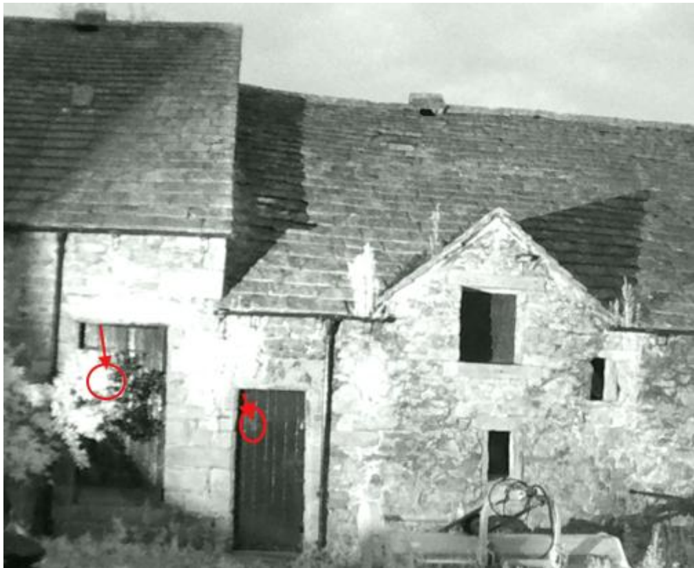
Image 3.2 Emergence point of 1 brown long-eared bat (front door access to loft - left of photo) on 25 th July and 2 brown long-eared bats on 29 th August.
