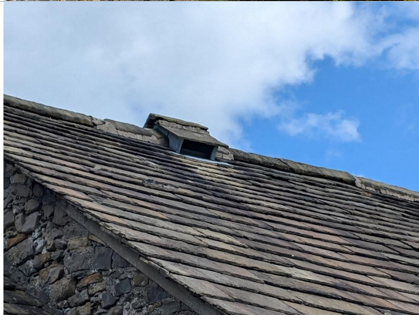
Photo 6. Close up of air vents.
