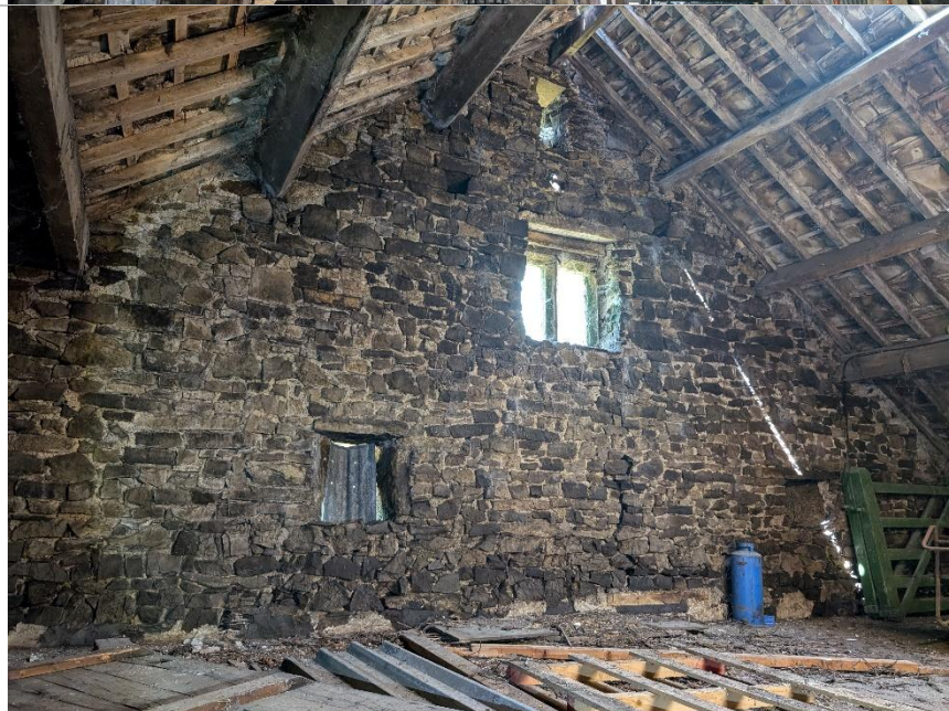
Photo 8. Internal view of west gable wall.
