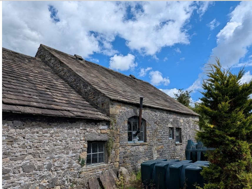
Photo 5. Rear (south) elevation of former stables.
