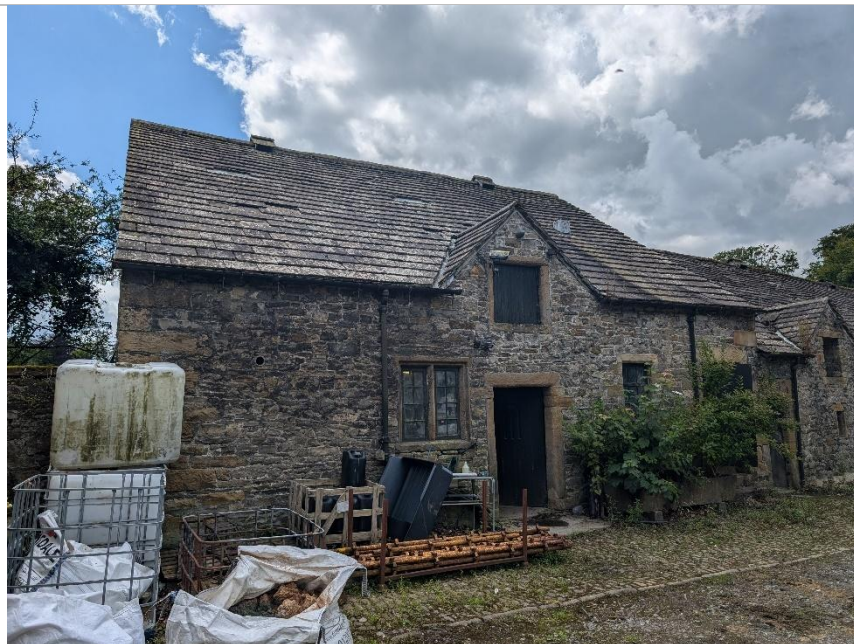
Photo 2. Front elevation of former stables.
