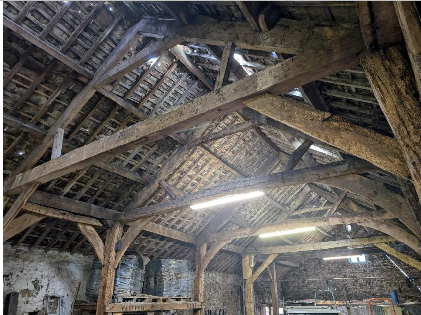
Photo 7. Roof framework of aisled barn (with lights).
