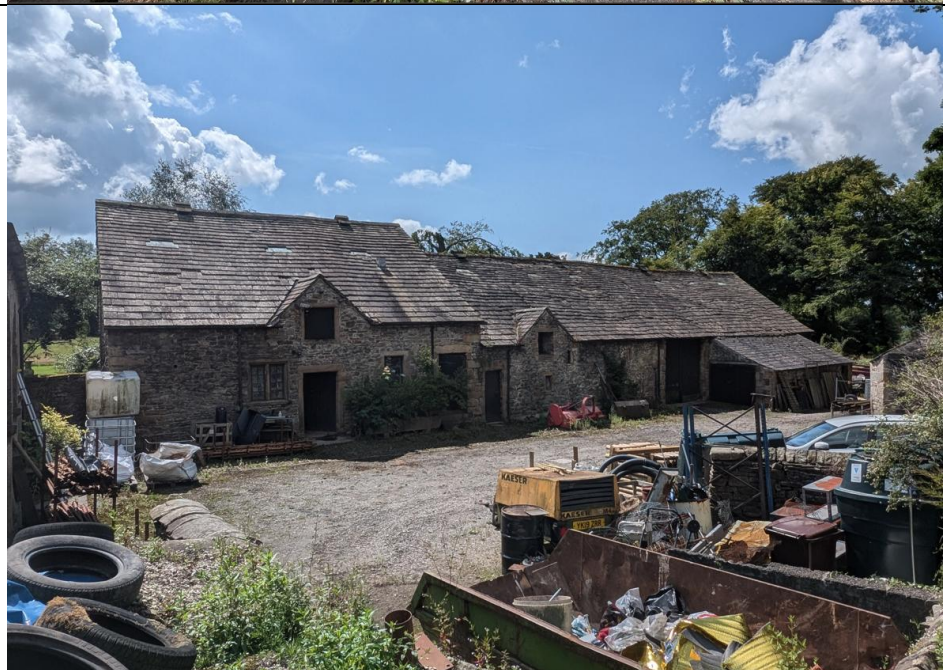
Photo 4. Aisled Barn and yard.
