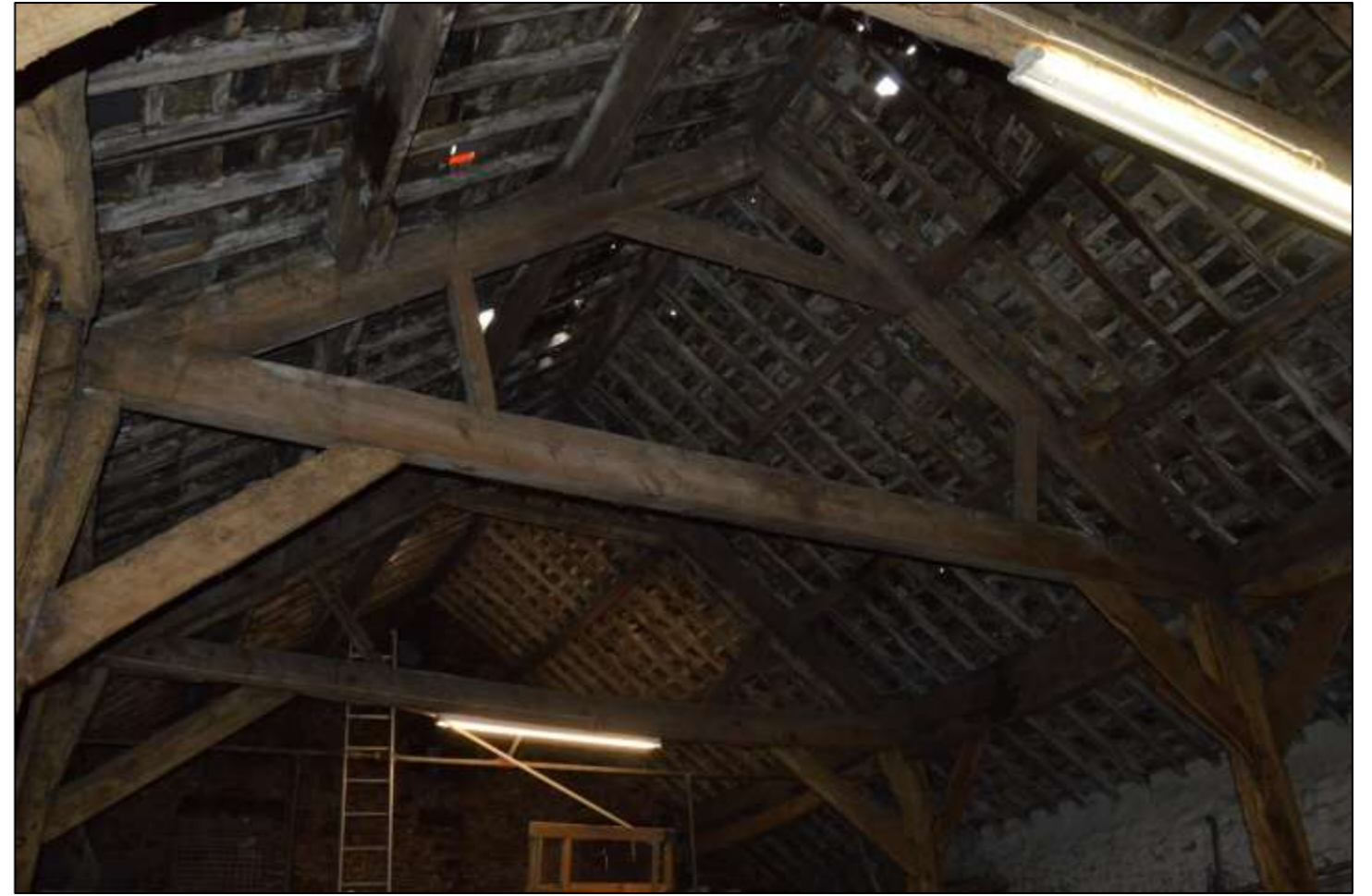
PL62: View of the roof structure over the eastern half of the barn.
