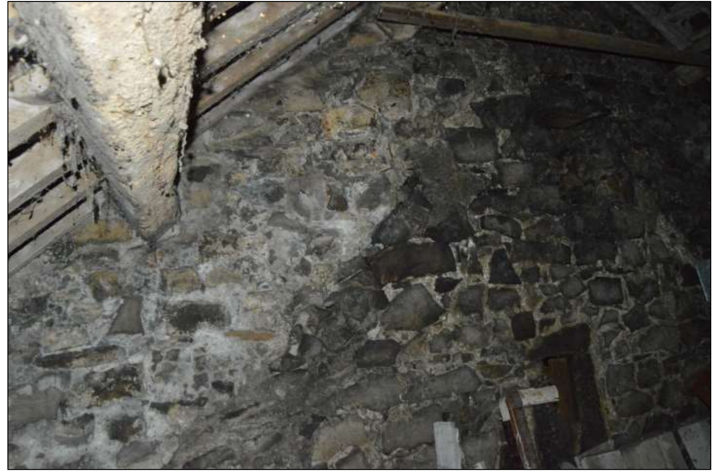
PL49: View of the west gable end within the first floor unit of the former stables. The outline of the gable end of the barn is visible.
