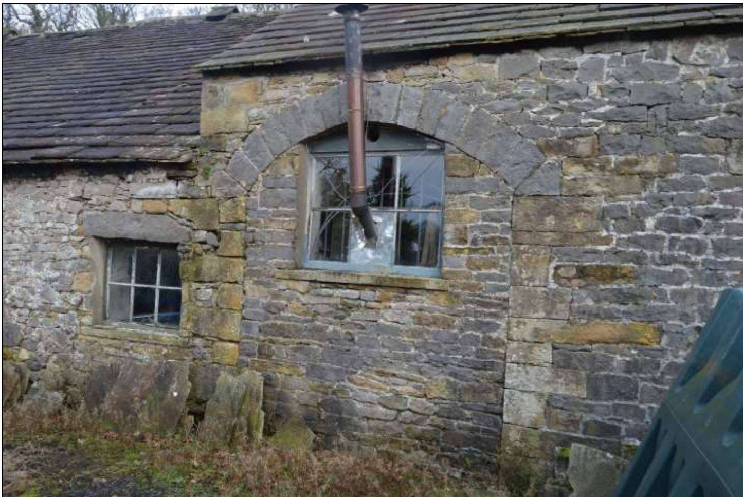
PL41: View of blocked up cart entry to the south facing elevation of the former stables, with inserted window.
