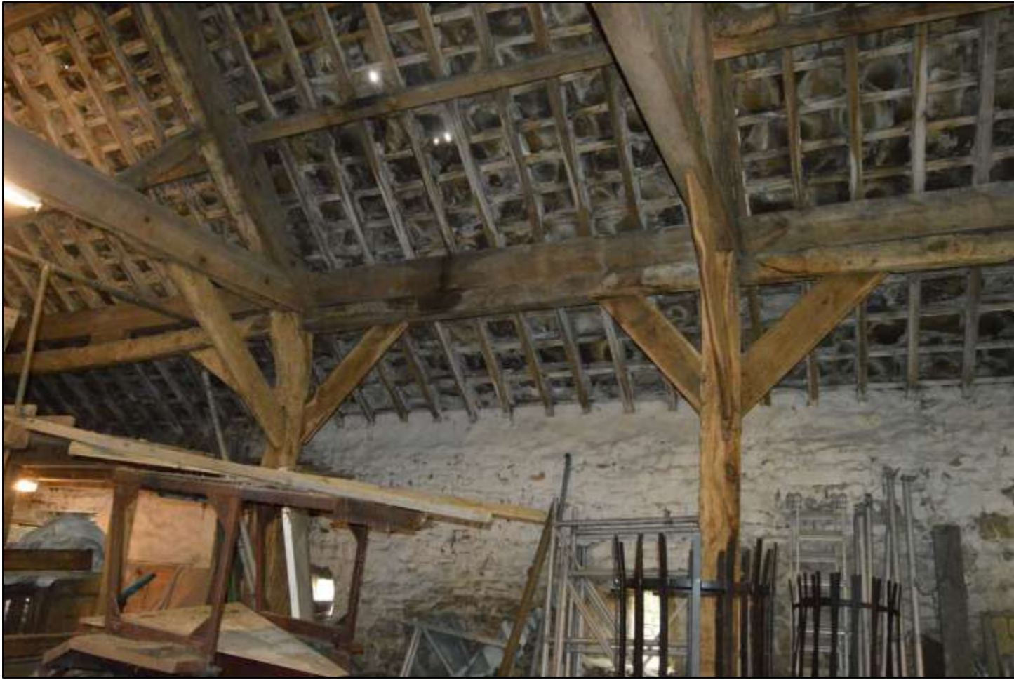
PL69: View of arcade posts and braces to the south side of the barn.
