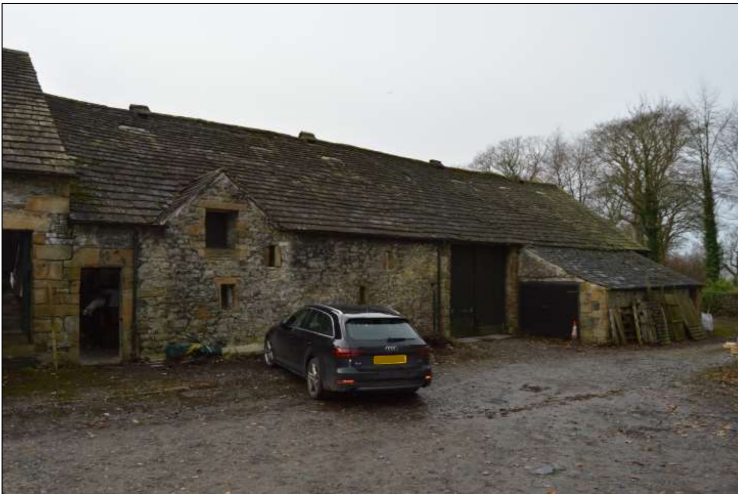
PL28: View of the north facing elevation of the barn.
