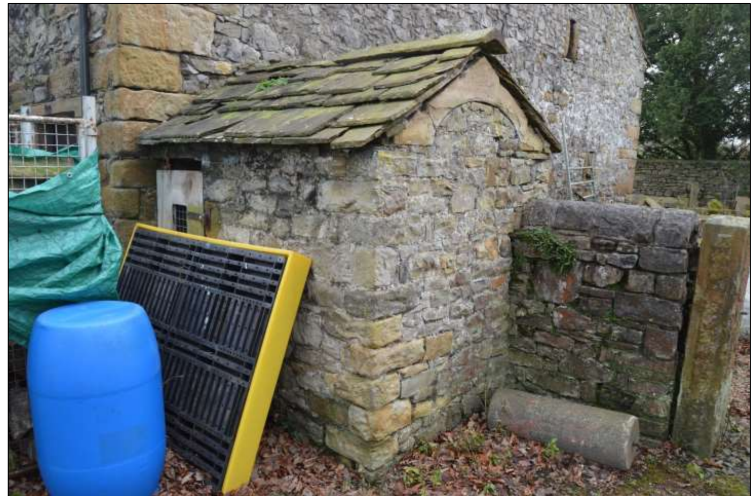
PL38: View of the former privy to the north west corner of the east gable end.
