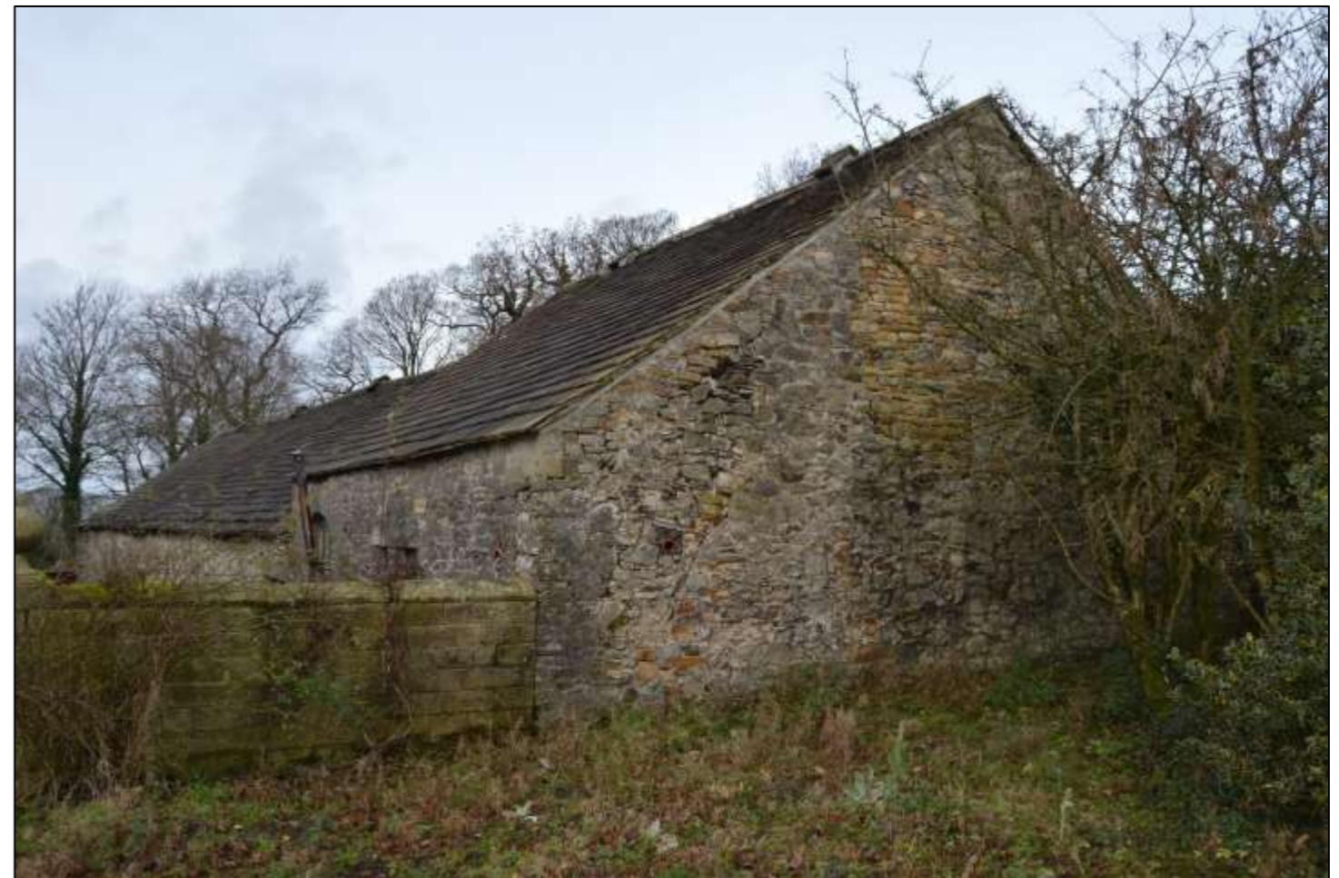
PL42: View of the former stable and barn from the south east.
