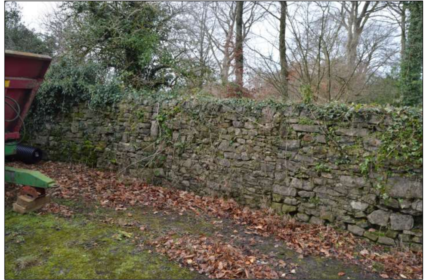
PL10: View of stone boundary wall located to the west of the barn, where the new site access is proposed.
