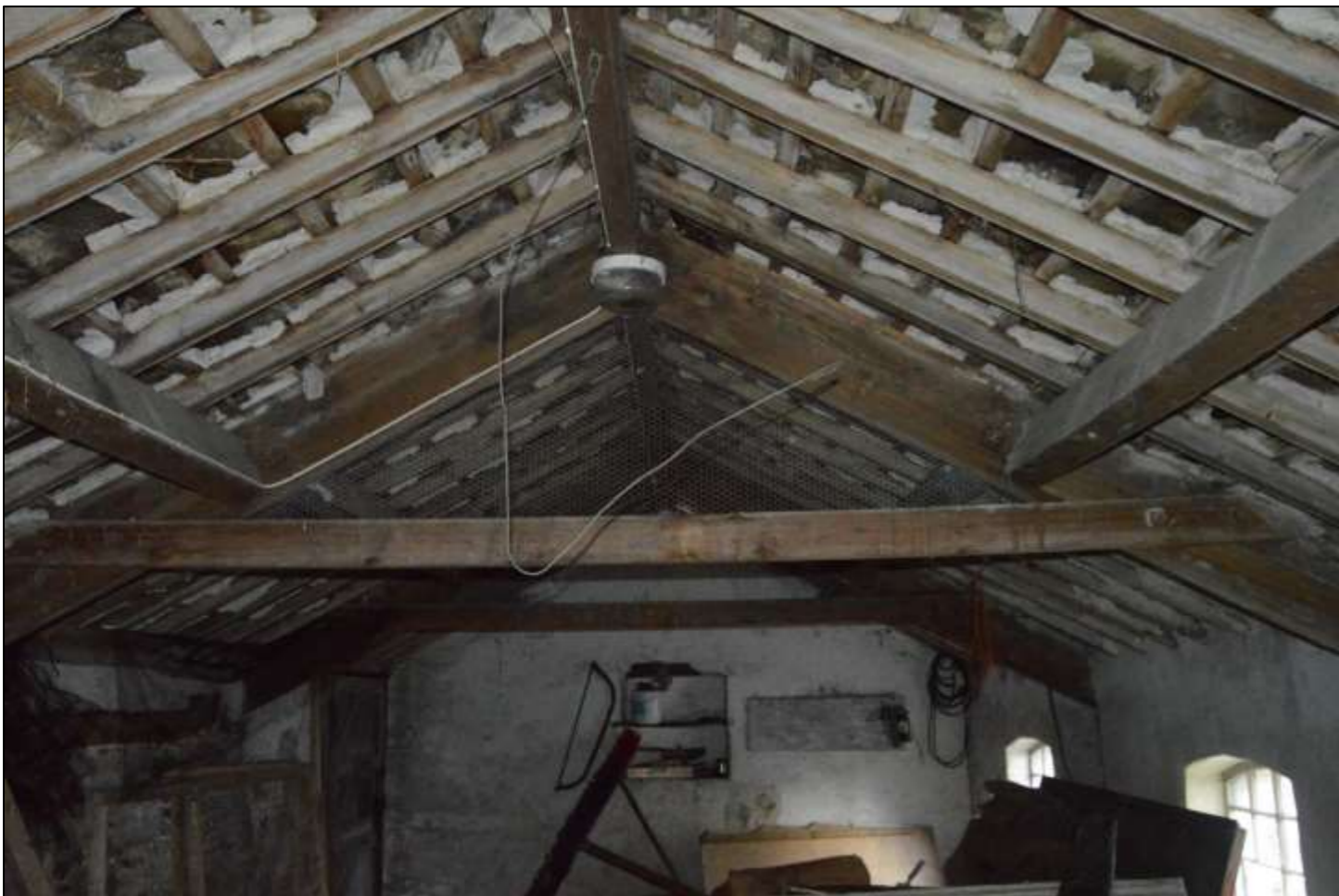
PL75: View of the existing timber roof structure to the former cart shed / granary from the north.
