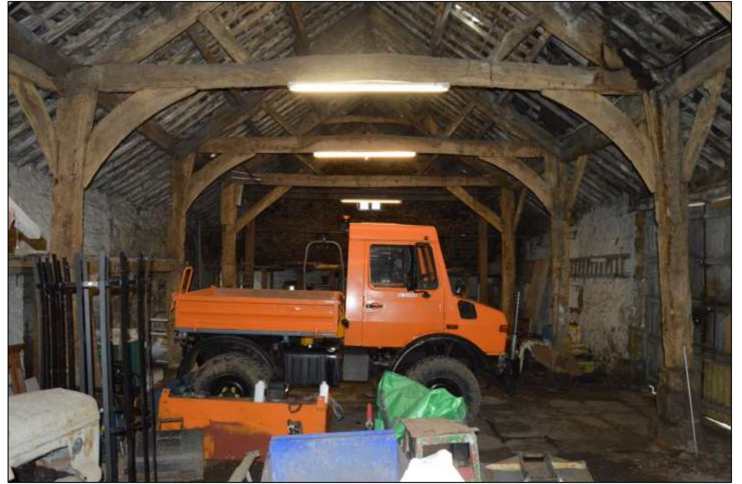
PL58: View west within the barn.
