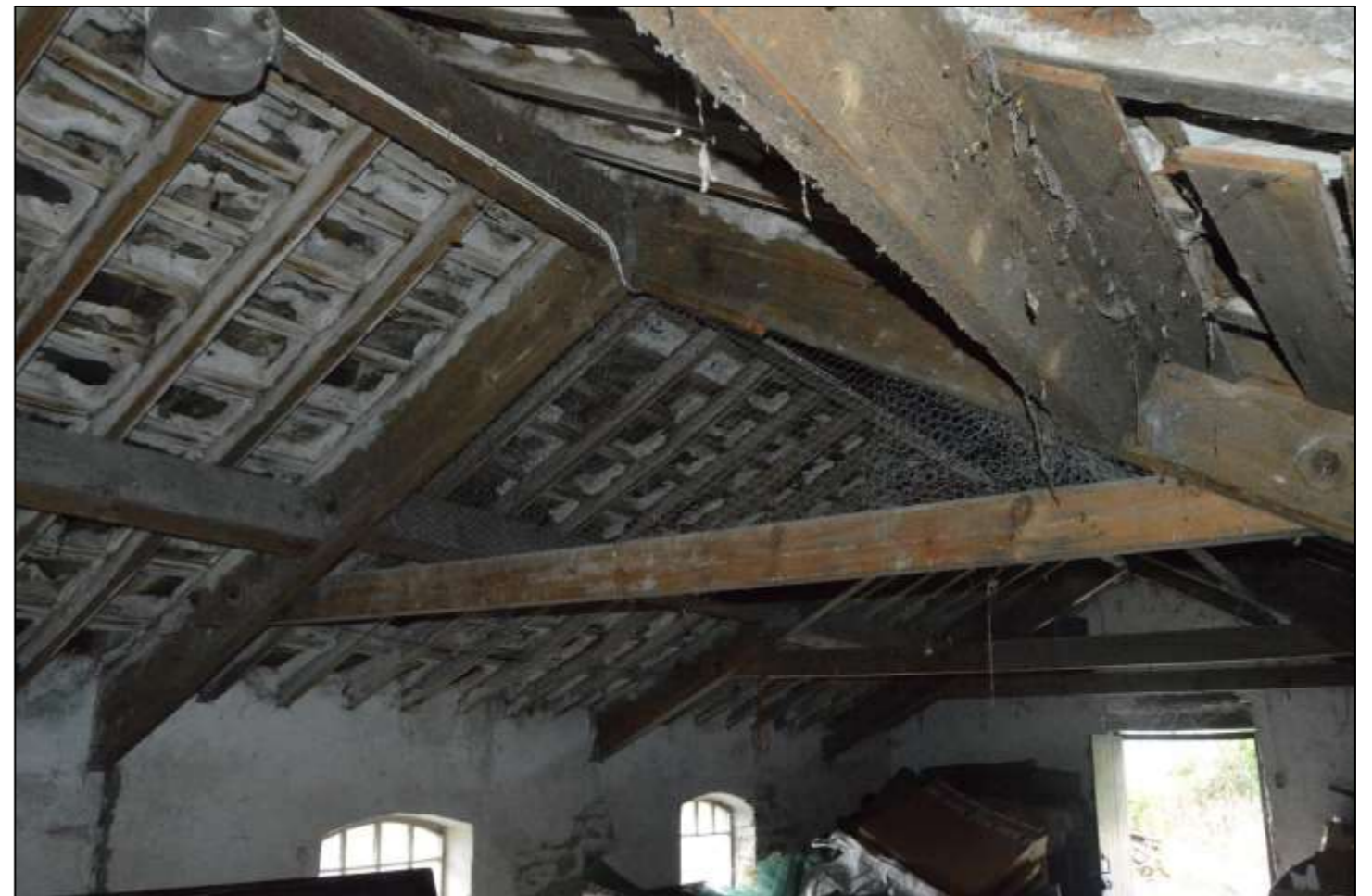
PL76: View of the existing timber roof structure to the former cart shed / granary from the south.
