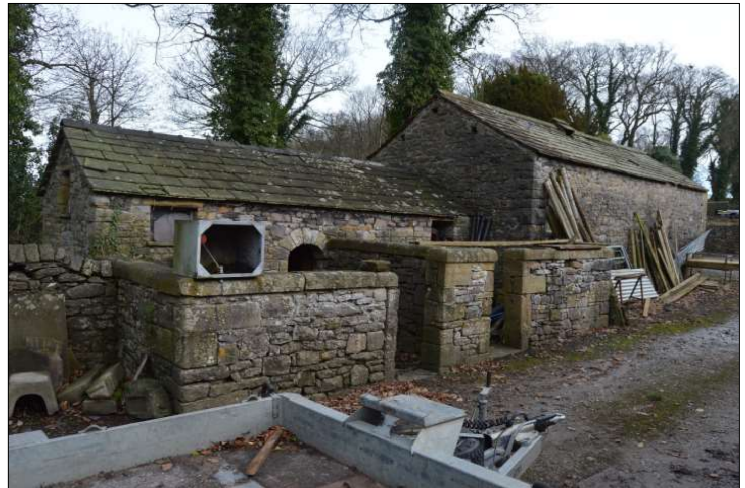
PL08: View of former stone built piggery located adjacent to the stone outbuilding.
