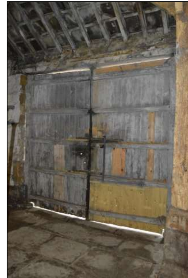
PL64: View of the harr-hung doors to the north elevation cart entry.
