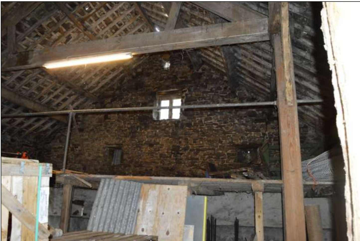
PL63: View of the west gable end and hay loft.
