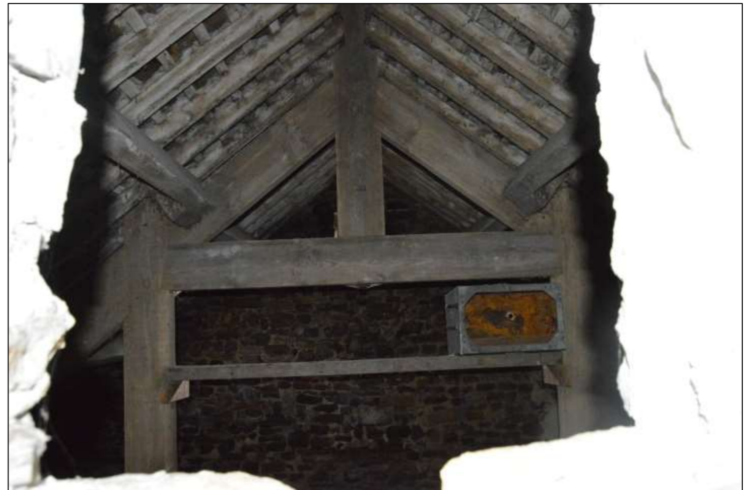
PL51: View into the first floor hay loft of the barn which was not accessible at the time of our site inspection.
