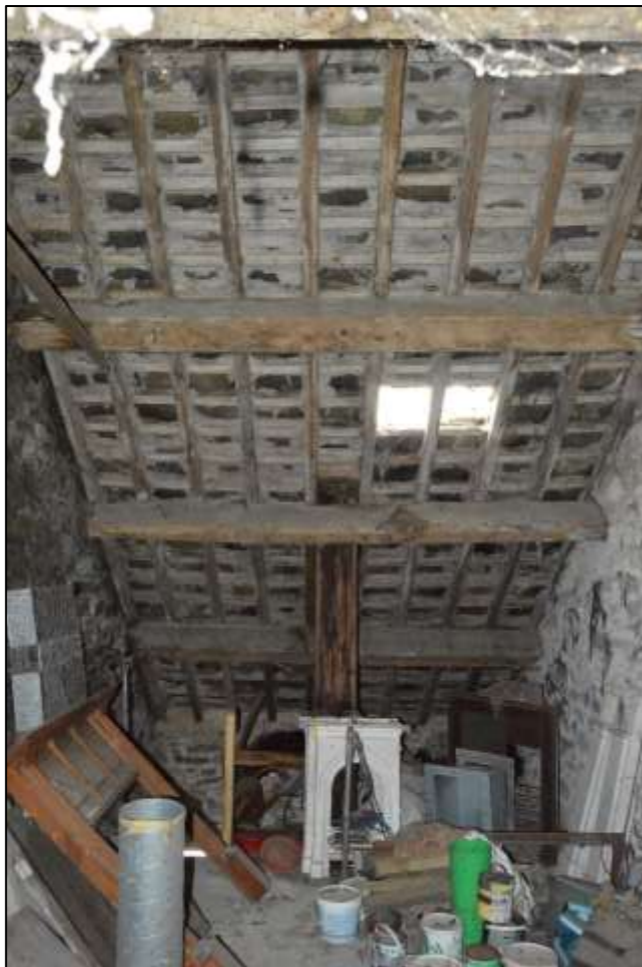
PL50: View of the roof structure to the north roof slope over the first floor unit of the former stables.
