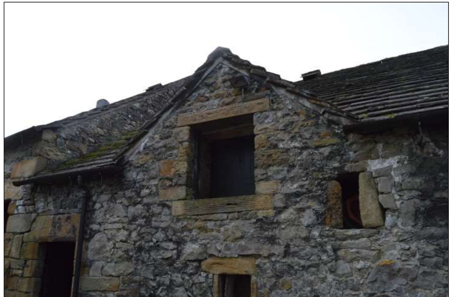
PL29: View of 19 th century pitching hole with gablet to the north facing elevation of the barn.
