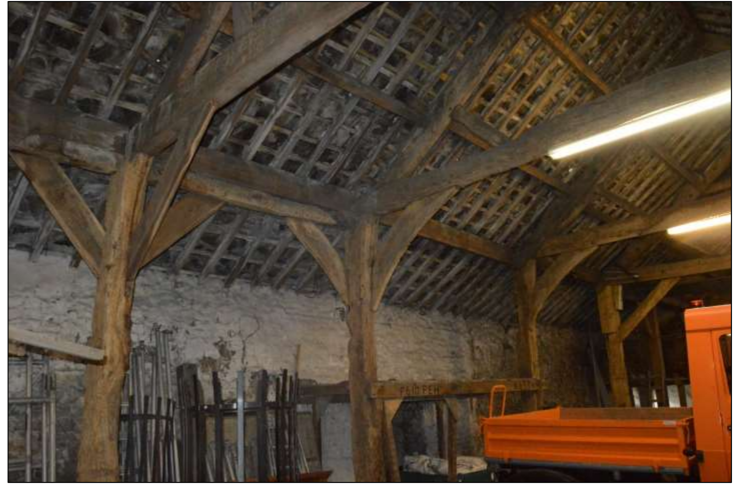
PL70: View of arcade posts and braces to the south side of the barn.
