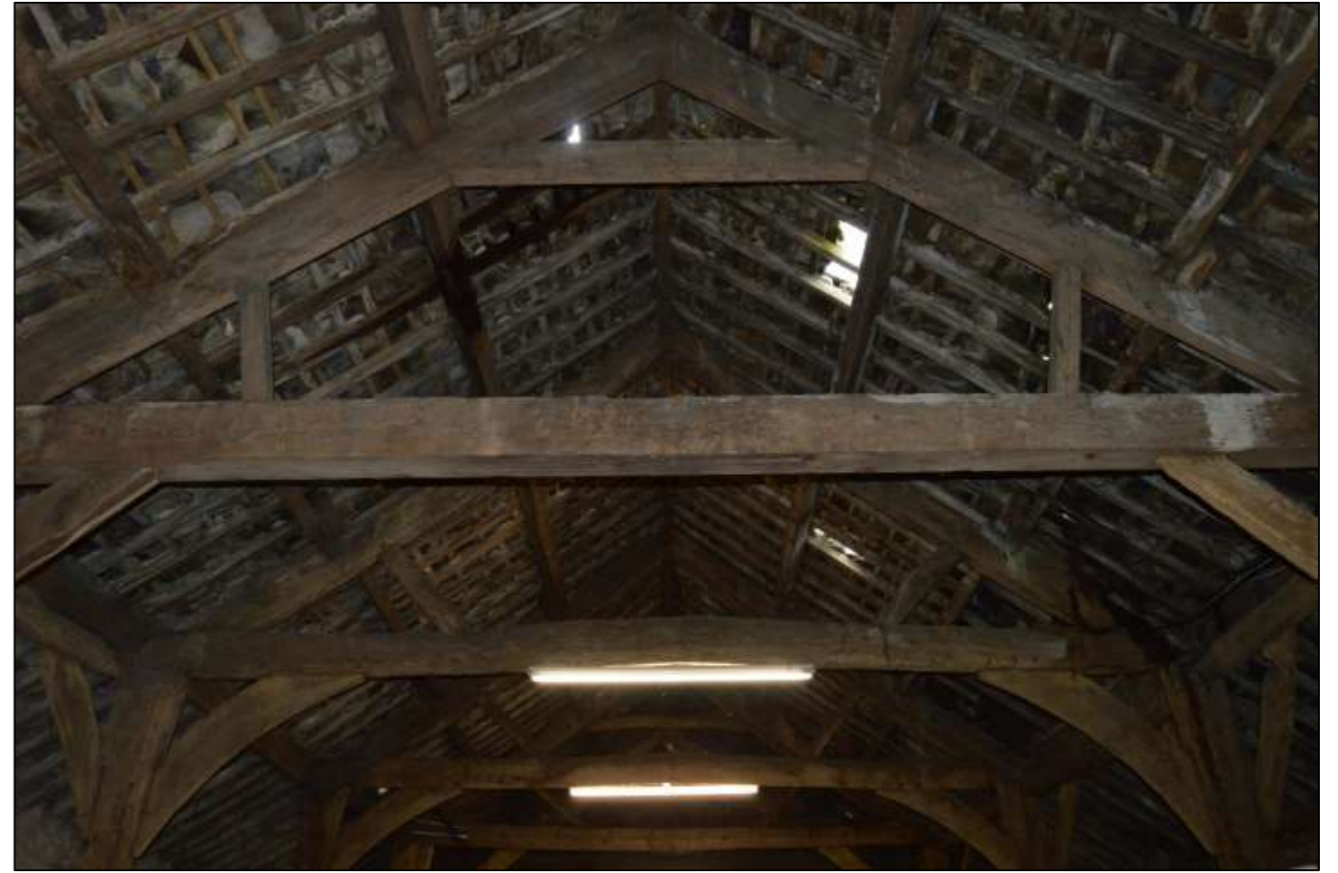
PL66: View of the roof structure over the eastern half of the barn.
