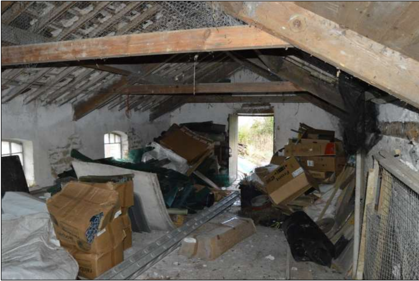
PL73: View north to the first floor of the former cart shed / granary.
