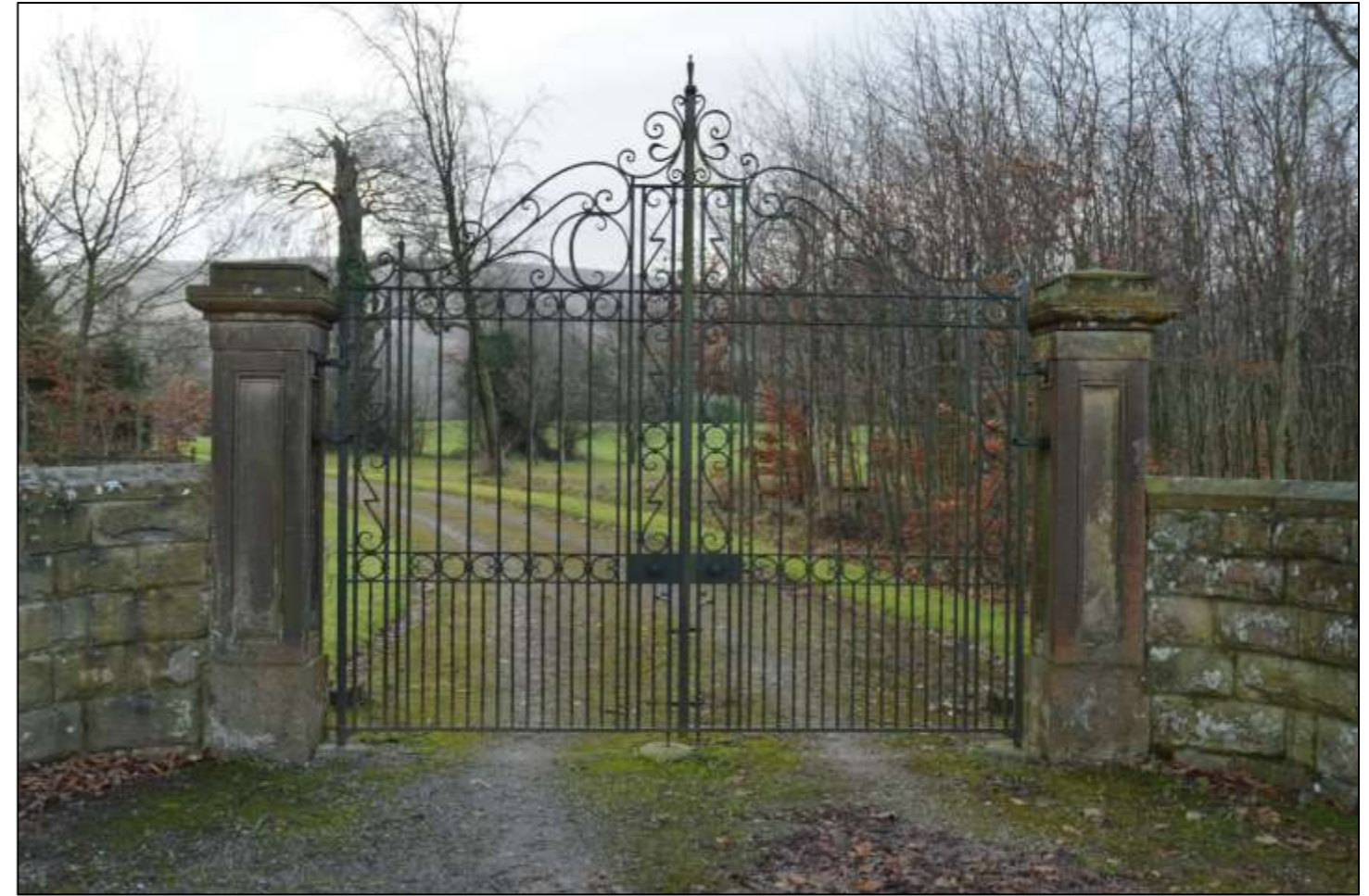
PL14: View of the existing stone gate posts and gates present to the existing site access to Downham Hall.
