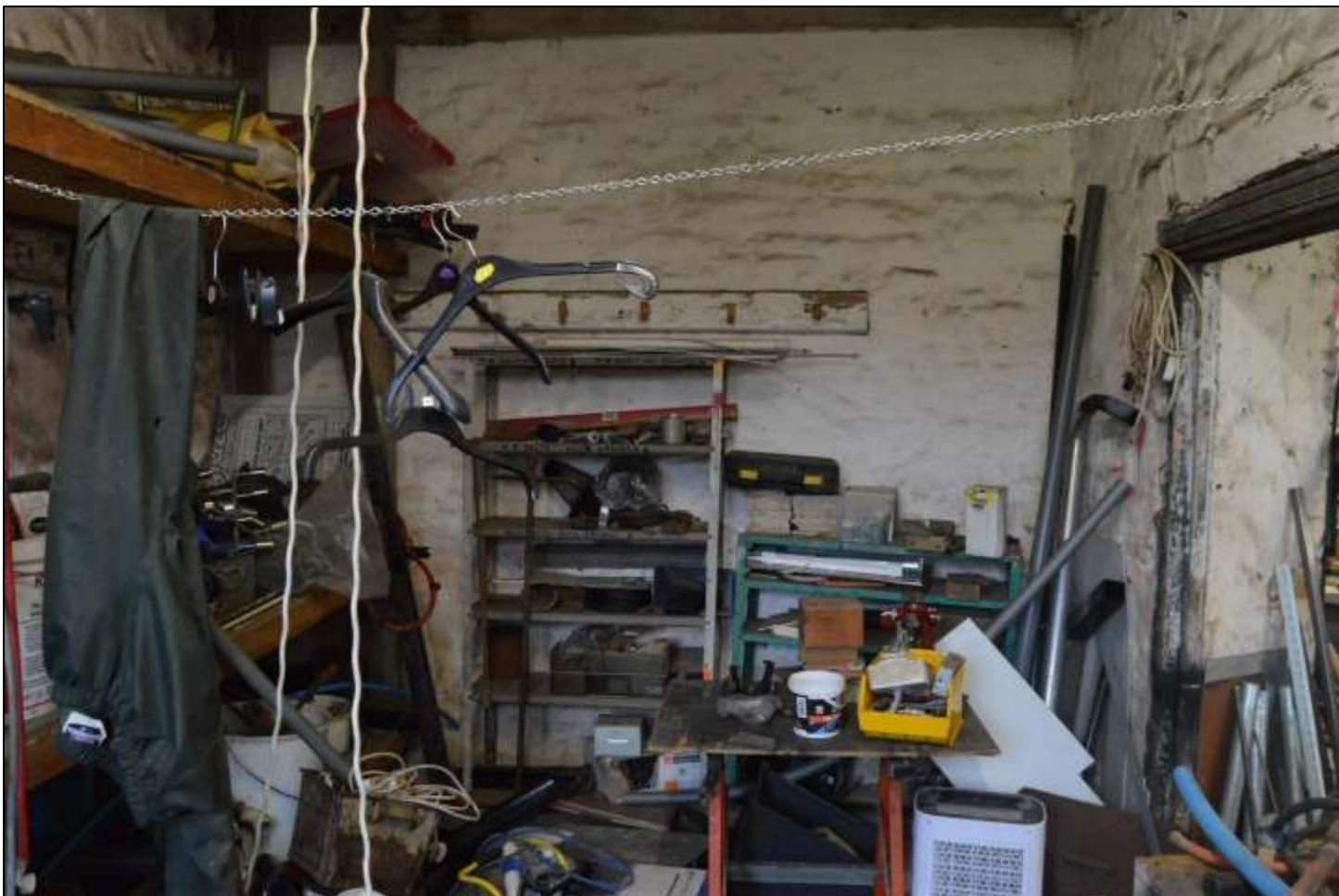
PL45: View north within the south west unit to the ground floor of the former stables.
