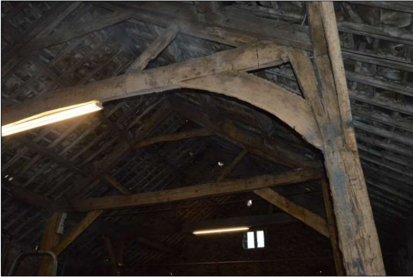
PL65: View of the roof structure over the western half of the barn.
