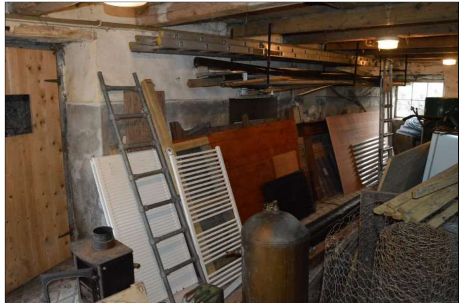
PL56: View east within the east shippen of the barn.
