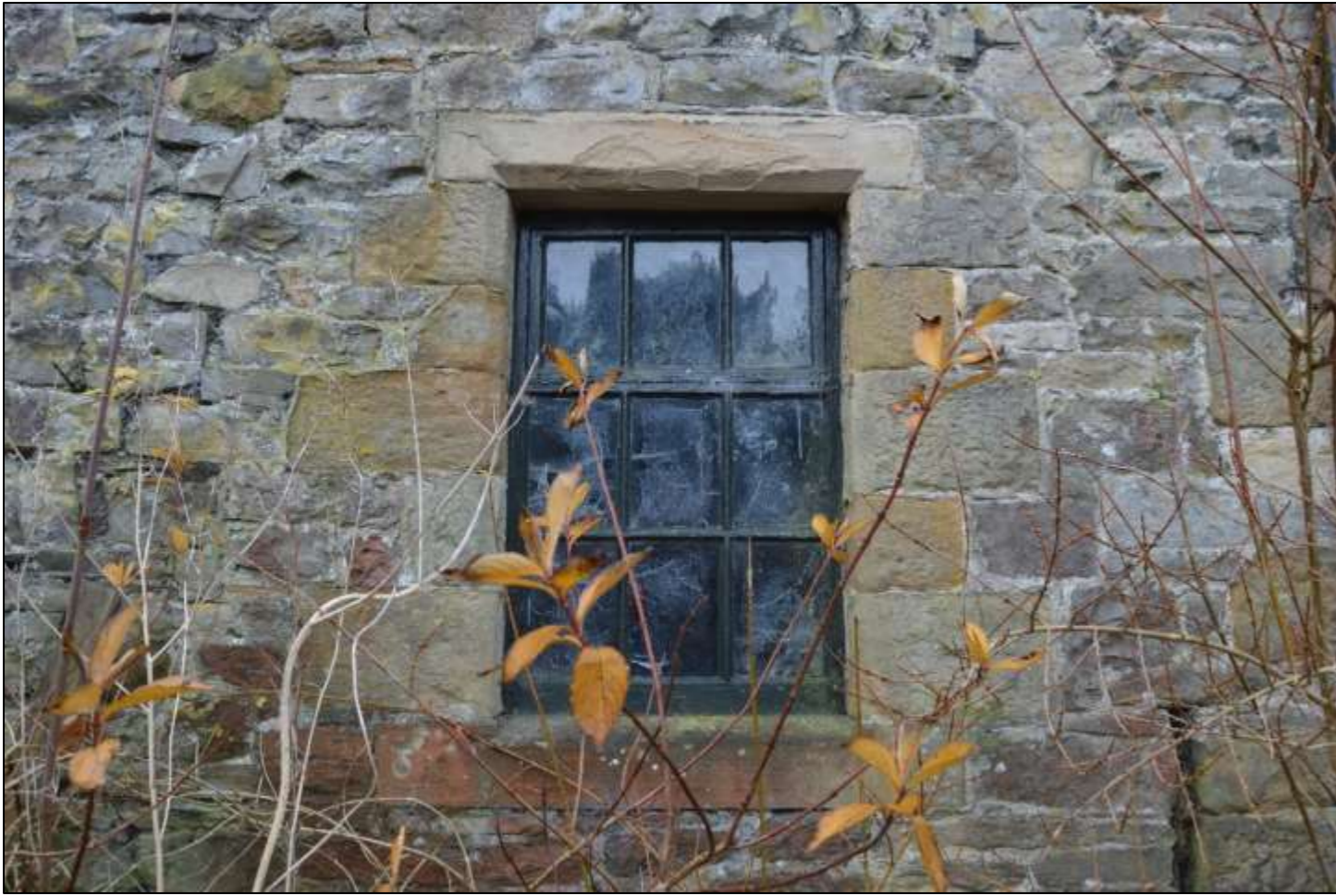
PL25: View of rebated window to the north facing elevation of the former stable with chamfered stone head and jambs.
