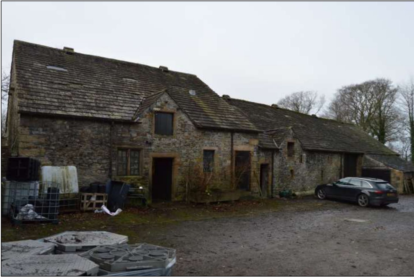
PL21: View of the former stable and barn from the north east.
