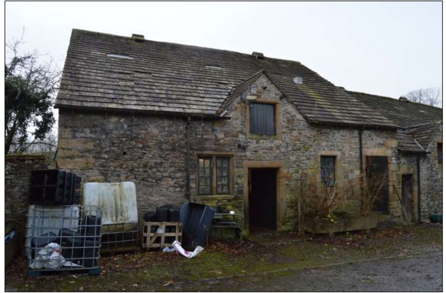
PL22: View of the north facing elevation of the former stables from the north east.
