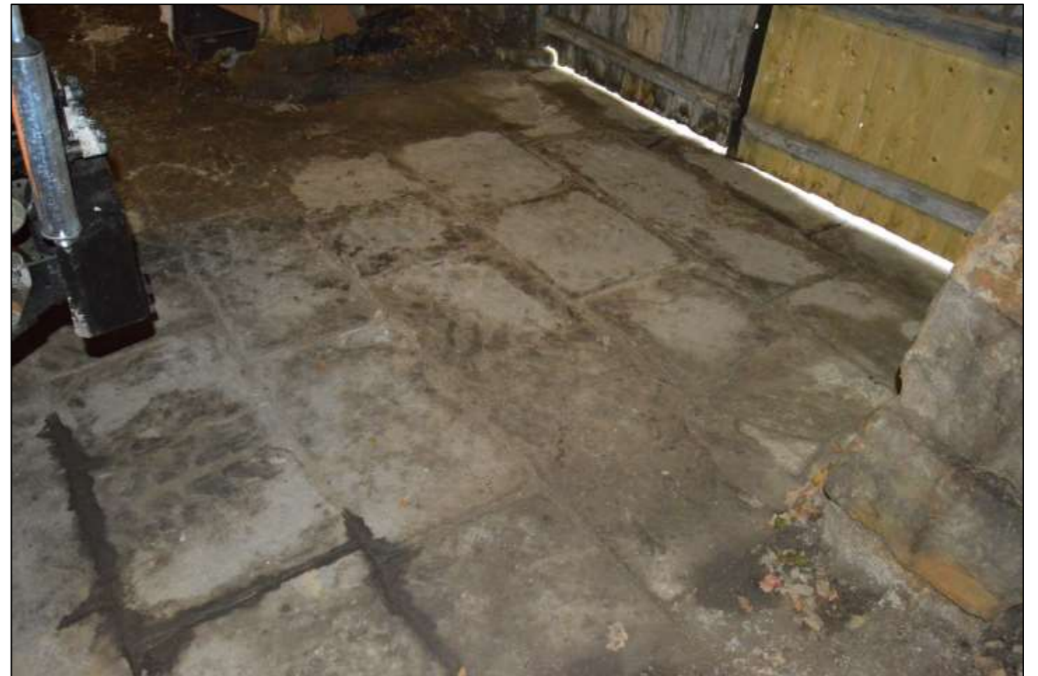
PL60: View of the stone flags adjacent to the barns cart entry.
