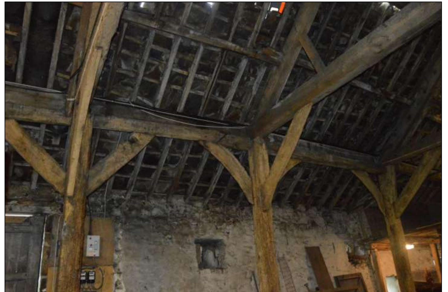
PL68: View of the arcade posts and braces adjacent to the east side of the north cart entry.
