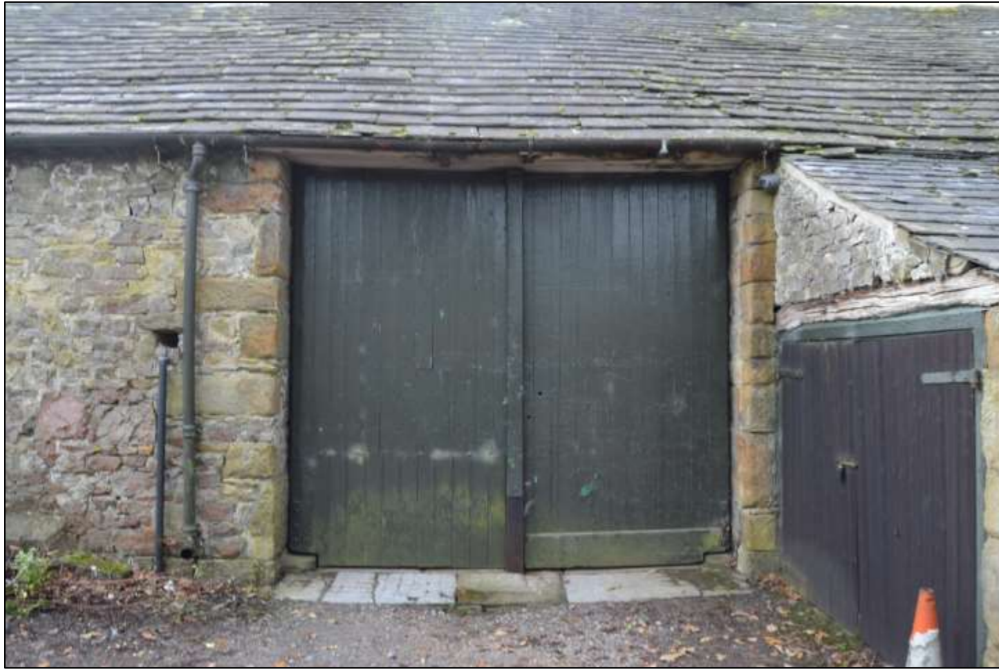
PL30: View of cart entry and harr-hung doors to the north facing elevation of the barn.
