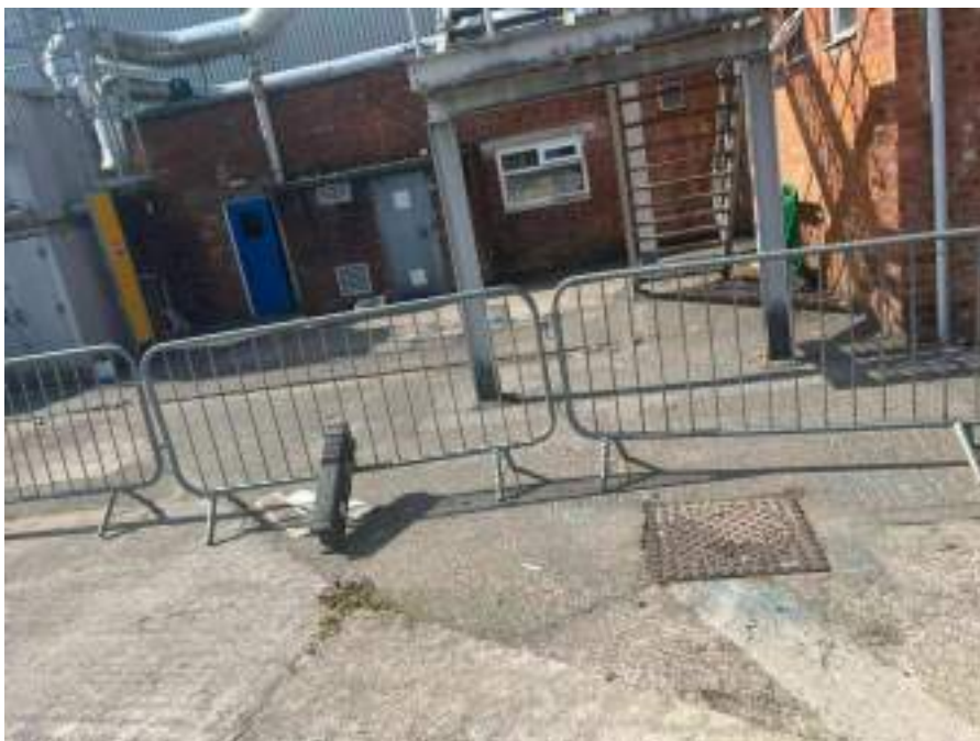
MH01X_D_13082025_0951_004.jpg, 00:00:30, 2.99 m Finish node, manhole, reference: MH02, MANHOLE LOCATED ADJACENT TO STAIRCASE
