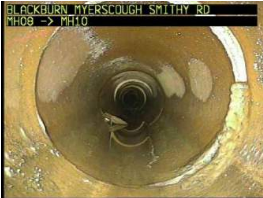
MH08X_D_14082025_1244_078.jpg, 00:03:33, 14.43 m Attached deposits, encrustation from 3 o'clock to 5 o'clock, 5% cross-sectional area loss
