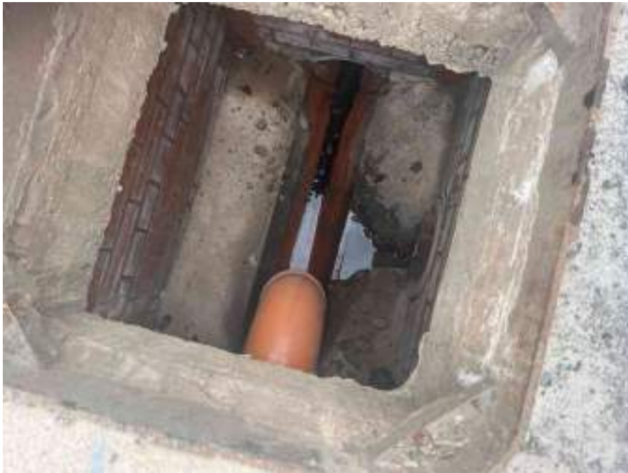
MH09X_D_14082025_1220_052.jpg, 00:00:27, 2.48 m Finish node, manhole, reference: MH08
