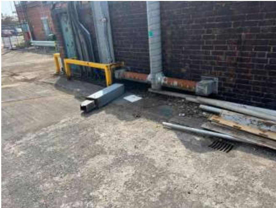
MH04AX_U_13082025_1217_039.jpg, 00:00:00, 0.00 m Start node, manhole, reference: MH04, MANHOLE LOCATED ADJACENT TO DUCTING
