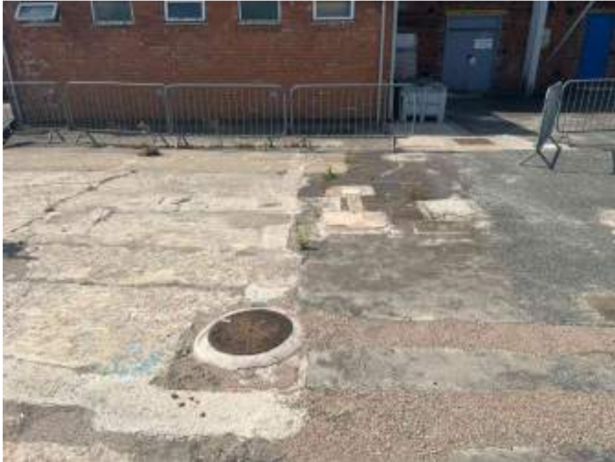
MH06X_D_13082025_1145_033.jpg, 00:00:00, 0.00 m Start node, inspection chamber, reference: MH06, IC LOCATED ADJACENT TO FILTER STORES
