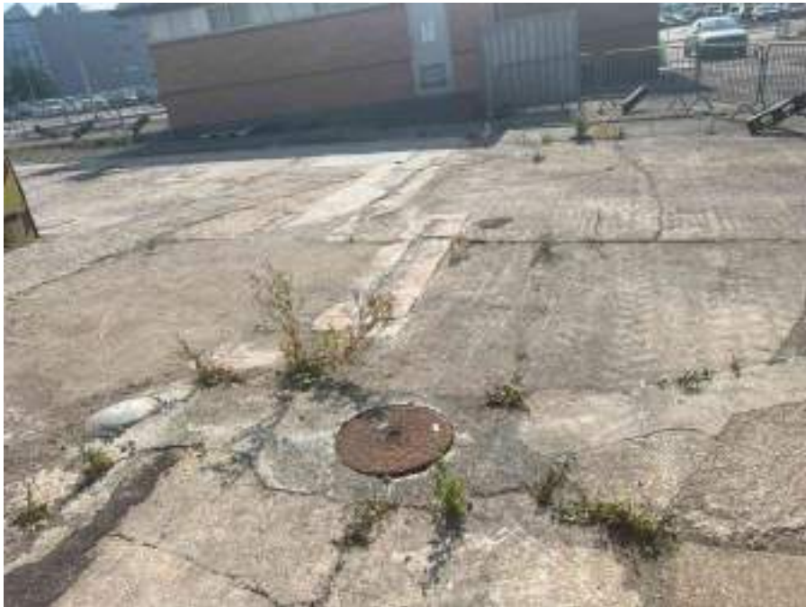
MH01AX_U_13082025_0954_006.jpg, 00:00:00, 0.00 m Start node, inspection chamber, reference: MH01, IC LOCATED ADJACENT TO STAIR CASE
