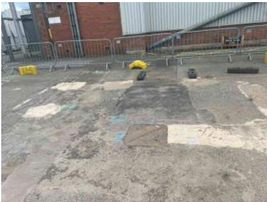
MH09X_D_14082025_1220_051.jpg, 00:00:27, 2.48 m Finish node, manhole, reference: MH08
