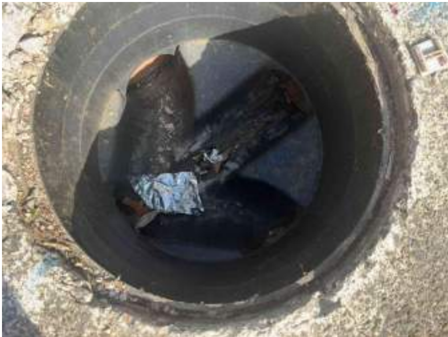
MH01X_D_13082025_0951_002.jpg, 00:00:00, 0.00 m Start node, inspection chamber, reference: MH01, IC LOCATED ADJACENT TO STAIRCASE
