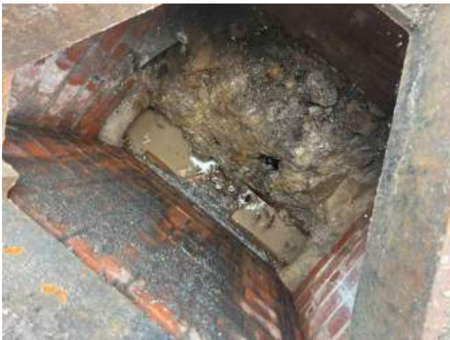
MH04BX_U_13082025_1225_046.jpg, 00:00:00, 0.00 m Start node, manhole, reference: MH04, MANHOLE LOCATED ADJACENT TO DUCTING
