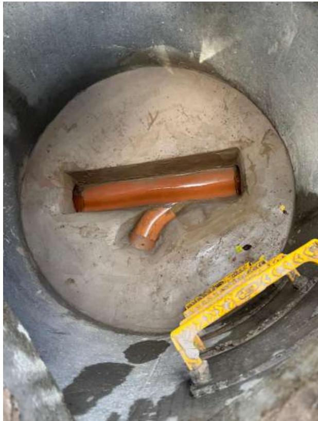
Photo 3 – as-built adopted combined sewer manhole in Crow Trees Brow
