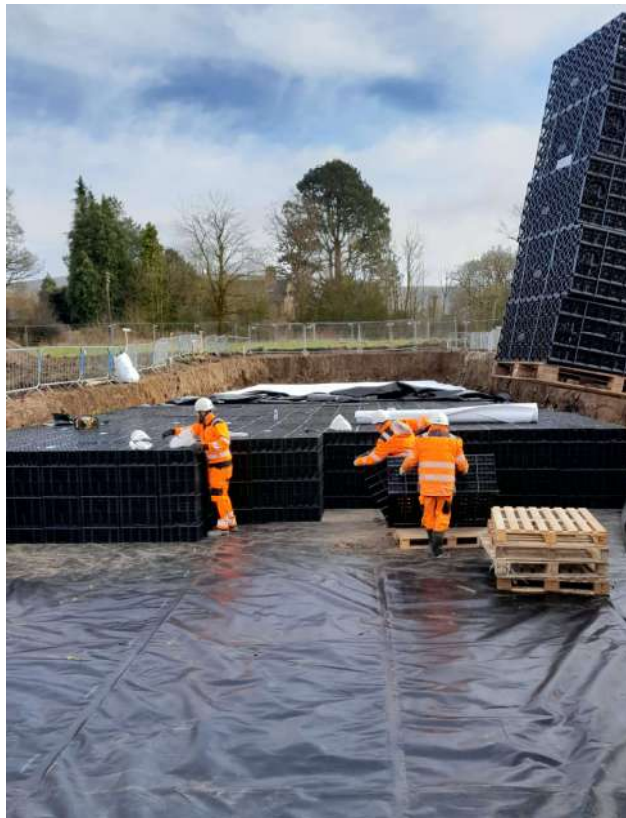
Photo 8 – installation of geomembrane and geocellular units
