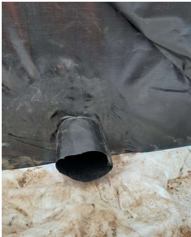
Photo 10 – geomembrane detail at inlet/outlet pipes
