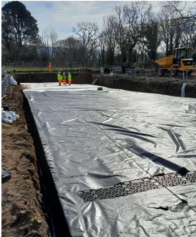
Photo 11 – geomembrane and geotextile installed over top of tank
