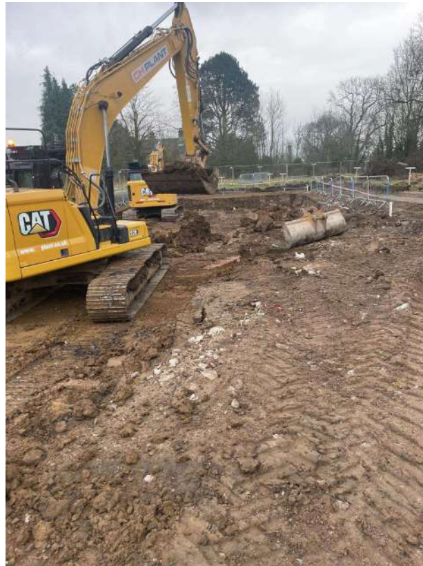
Photo 1 – excavation for geocellular attenuation tank
