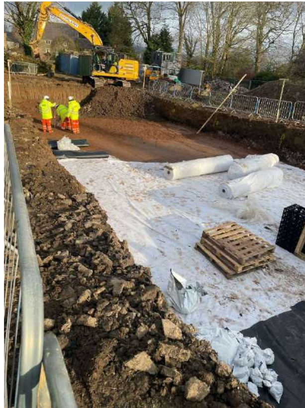
Photo 5 – installation of sand bedding course and geotextile protection fleece
