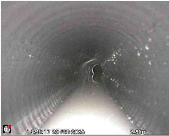
1, 00:00:29, 2.80 m General photograph taken at this point, line bending left without fitting
