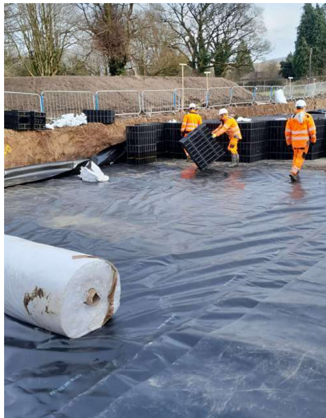
Photo 6 – installation of geomembrane and geocellular units
