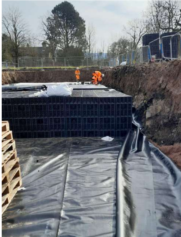
Photo 7 – installation of geomembrane and geocellular units
