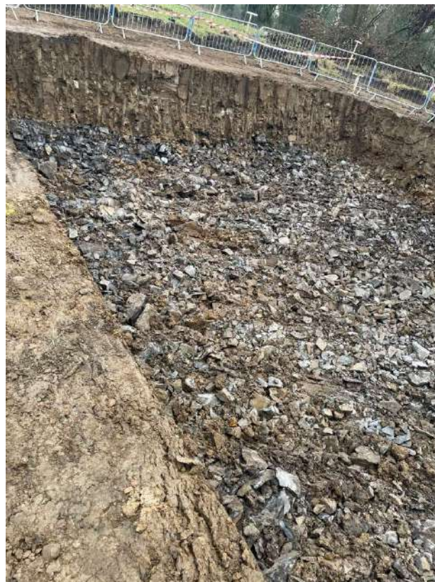
Photo 4 – excavation for geocellular attenuation tank
