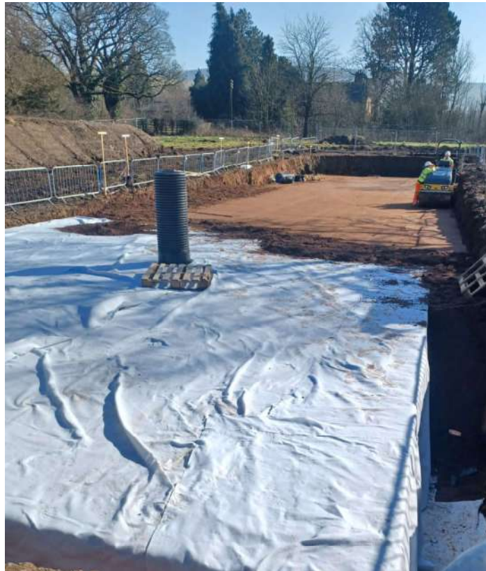
Photo 13 – installation of access turrets and sand backfill
