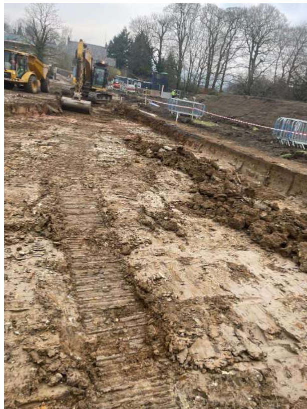
Photo 2 – excavation for geocellular attenuation tank
