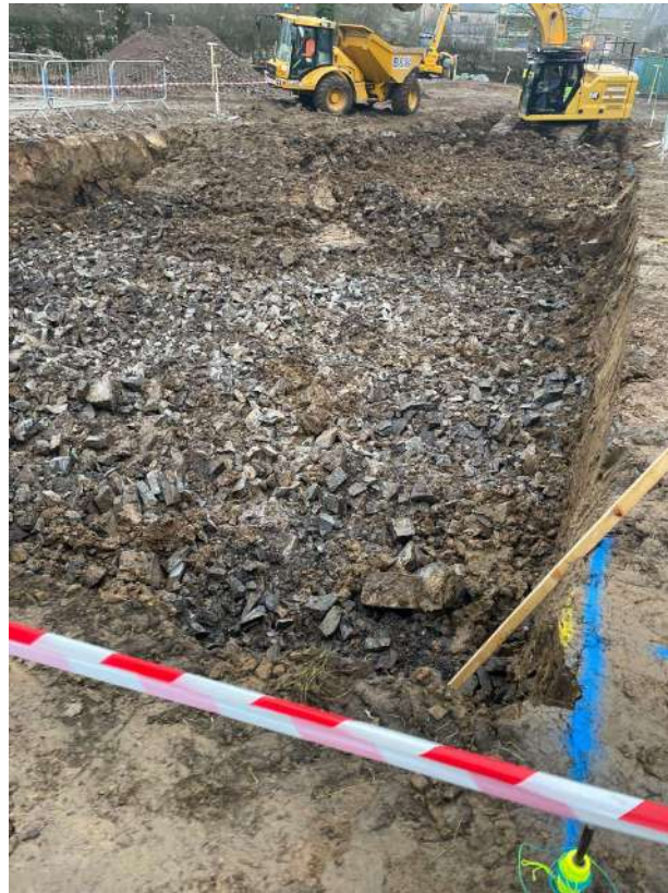
Photo 3 – excavation for geocellular attenuation tank
