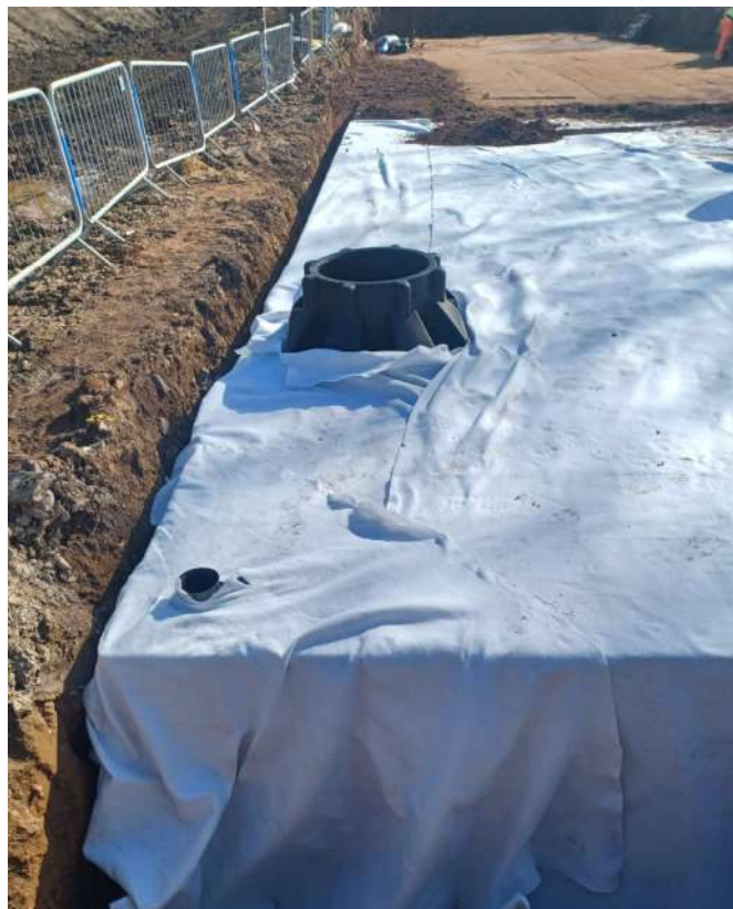
Photo 12 – installation of access units
