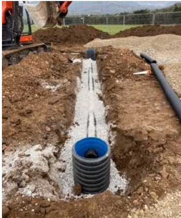
Installing drainage silt traps, Cheddar, Somerset
