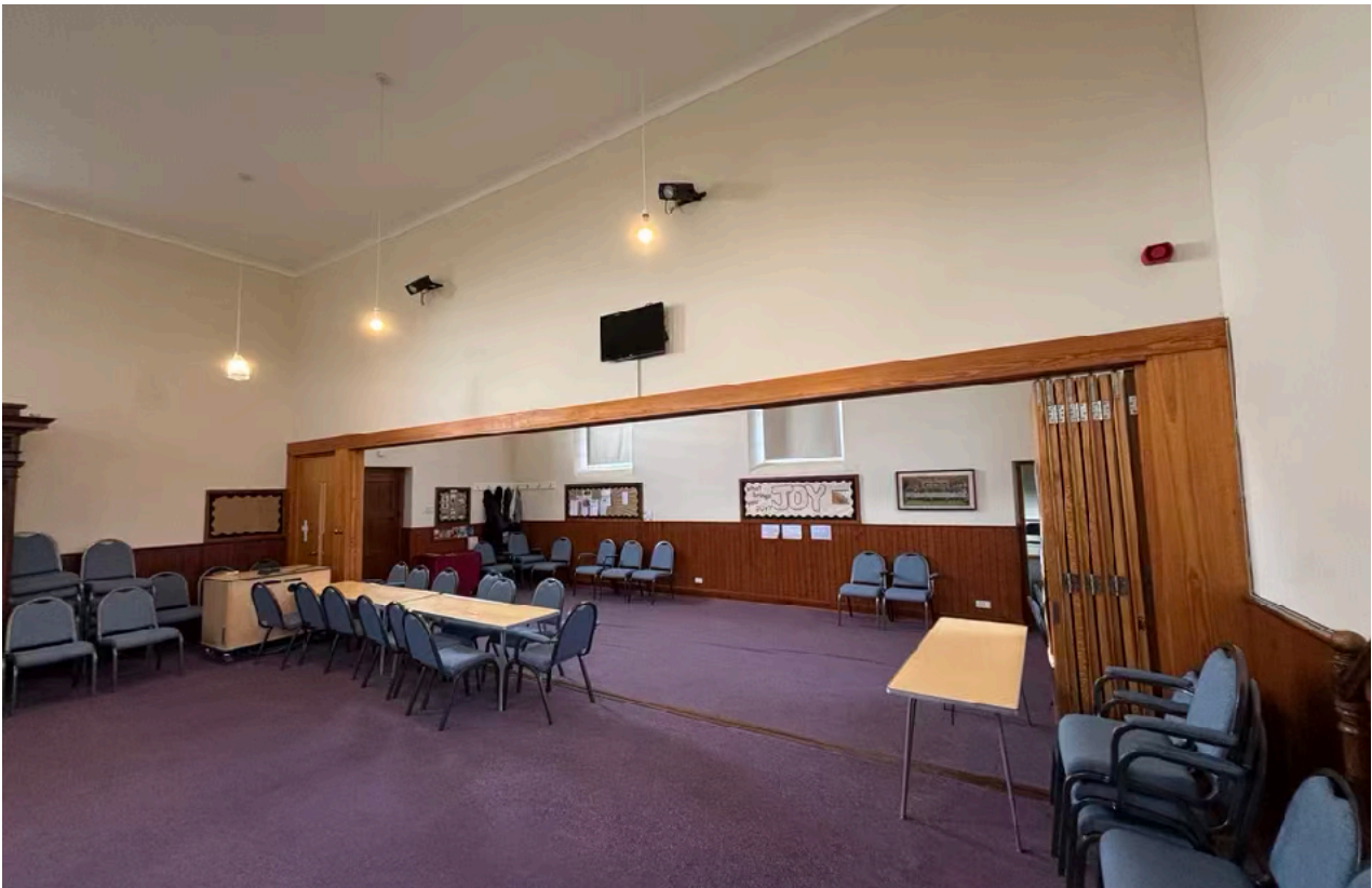
Figure 4: Location of the proposed first floor as seen from the southernmost room of main hall building.
