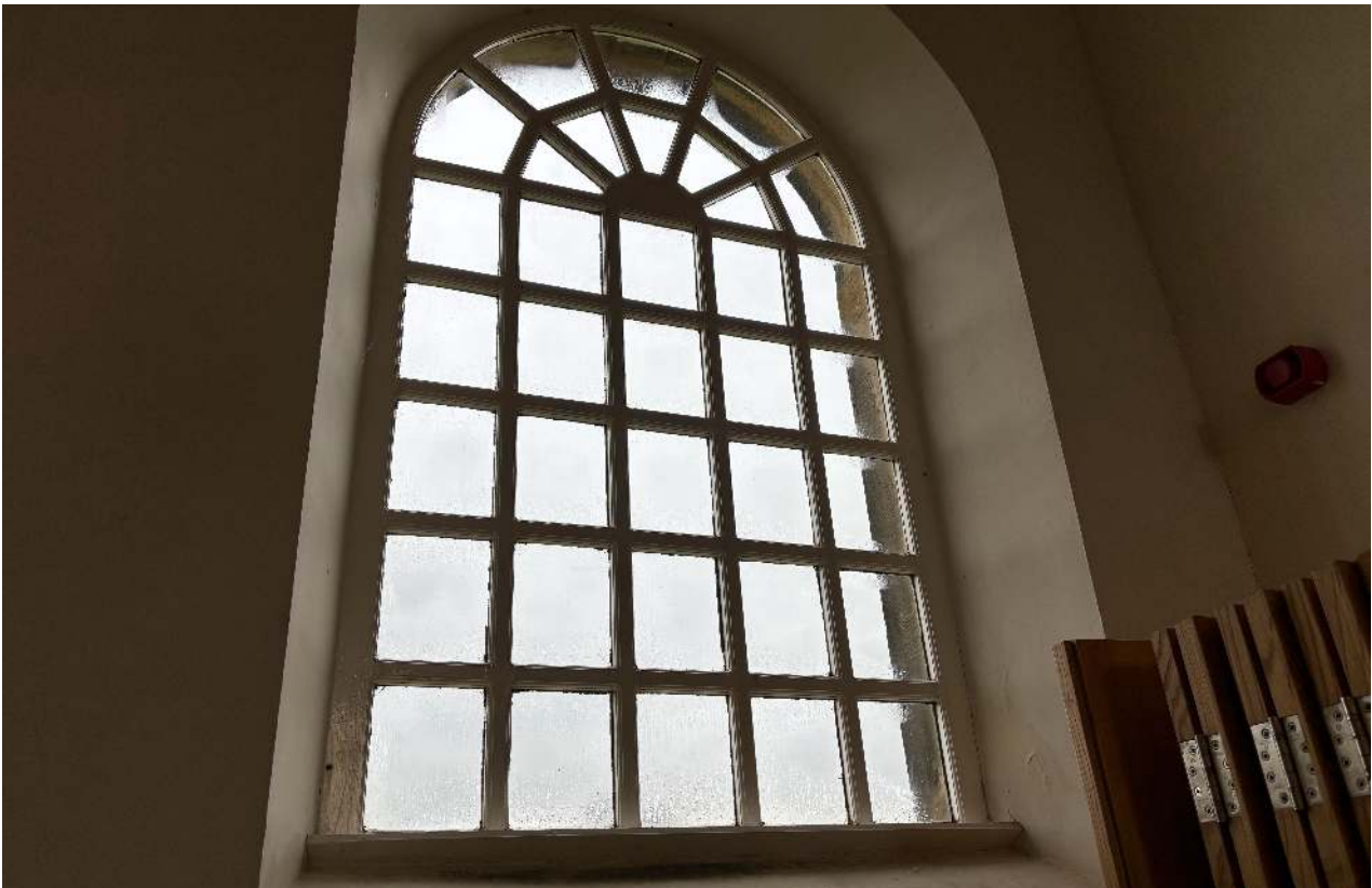
Figure 2: Typical window opening and frame.
