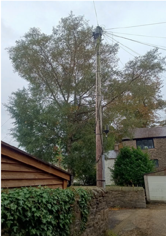
Picture showing protruding branch over lines.
