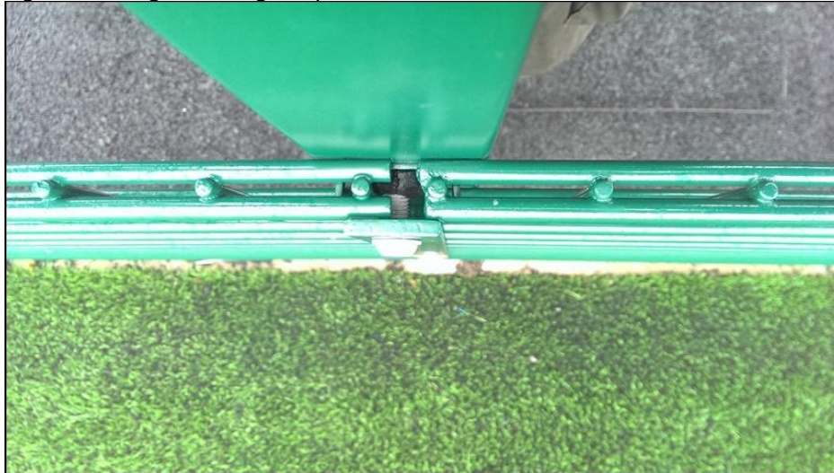
Figure 8: Image showing neoprene isolators
