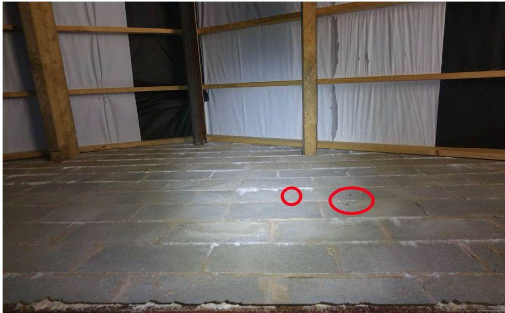
Location of bat droppings on interior wall
