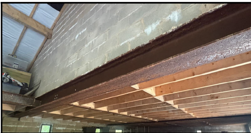
Internal wall at mezzanine level showing steel beams and timber joists.
