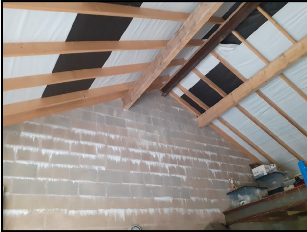
Internal view of west gable showing roof and wall construction.
