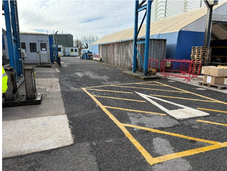
Photograph 3-1: Area of other developed land (u1b6) within Site 1 - Main Control Room (B2)
