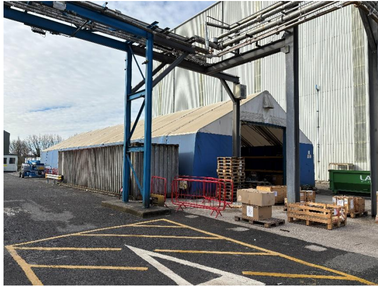
Photograph 3-3: The marquee tent (B1) located within Site 1 - Main Control Room
