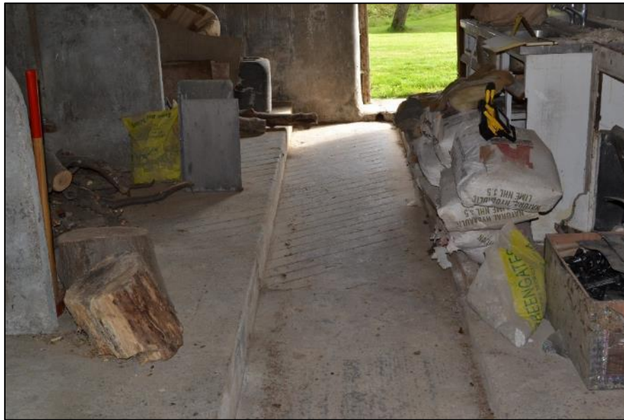
Plate 14. Ground floor, concrete dairy floor
