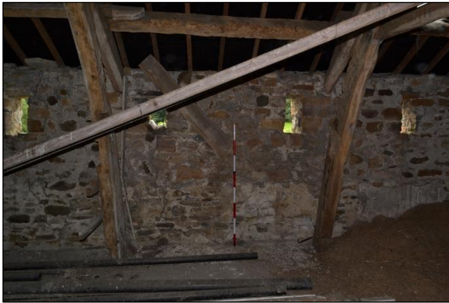
Plate 20. First floor south elevation and original crucks (scale 16m)
