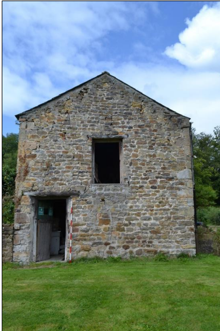
Plate 9. The east elevation (scale 2m)
