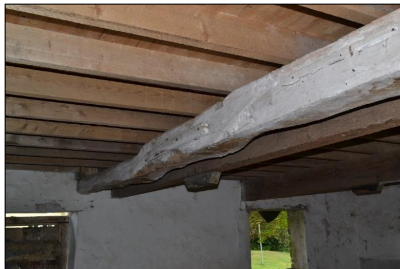
Plate 17. Showing original simple transverse joists
