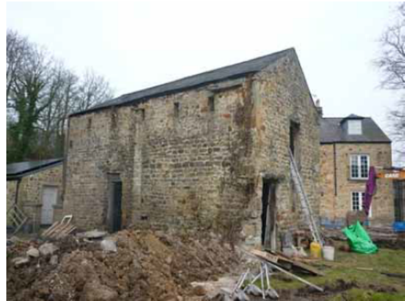
Photo 2: Rear of barn
