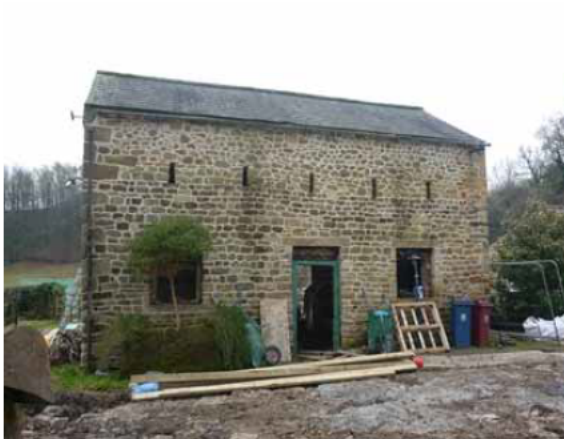
Photo 1: Front of barn
