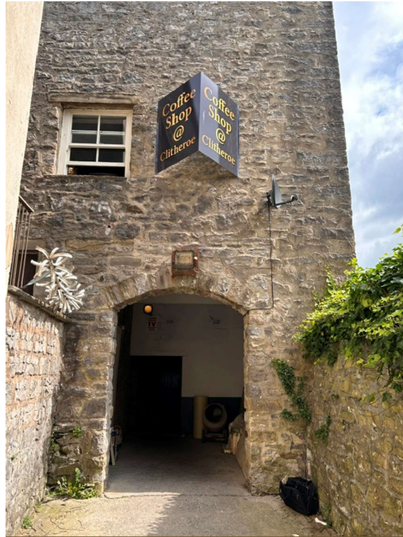
Access to the covered seating area from Lowergate car park
