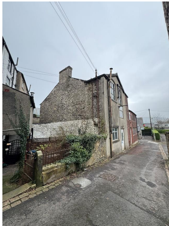
E6 – View of the NW Side Elevation and SW Front Elevation.
