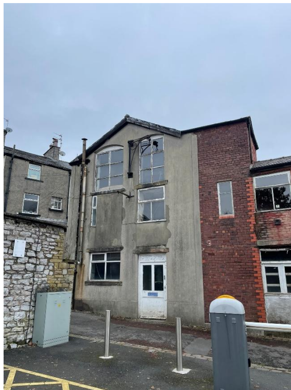
E8 – Principal Elevation showing infilled openings, render, and jib crane.
