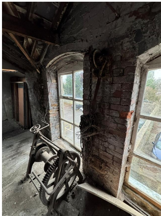
E10 – Internal Pulley and chain to be restored/ retained.
