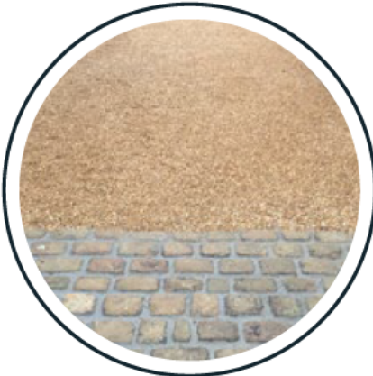
2 Permeable road surface
