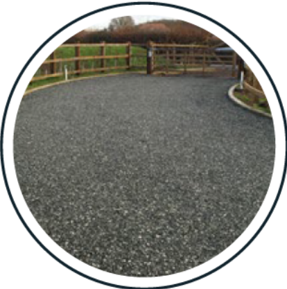
1 Tarmacadam access road
