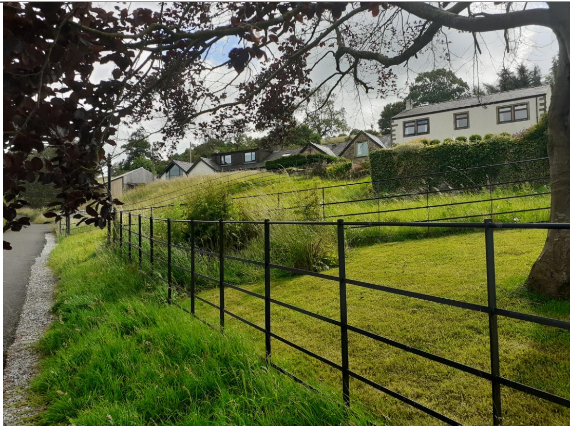
6 Gable features on Ribble View in stone viewed from the bridleway
