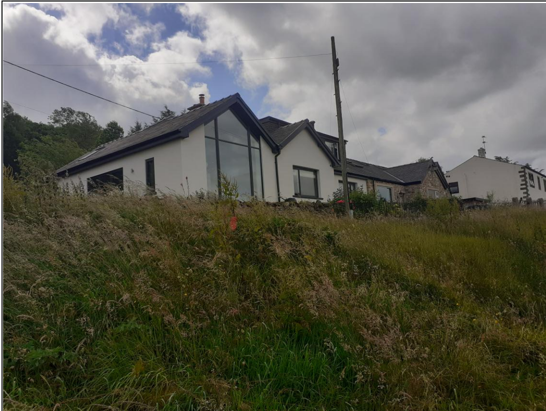
5. Gable feature on Ribble Dene. The height to the ridge on this gable is shown as 4.752m on the approved drawing, the main ridge is higher again. The height to the ridge on the gable of the proposed holiday accommodation 4.39m
