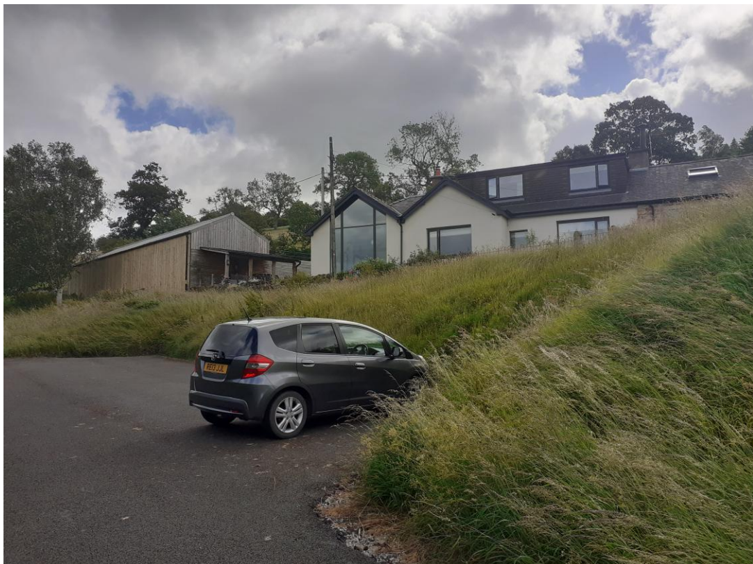
2. Ribble Dene looking east from the bridleway. Note glazed gable feature and timber clad outbuilding. The application site is behind these buildings
