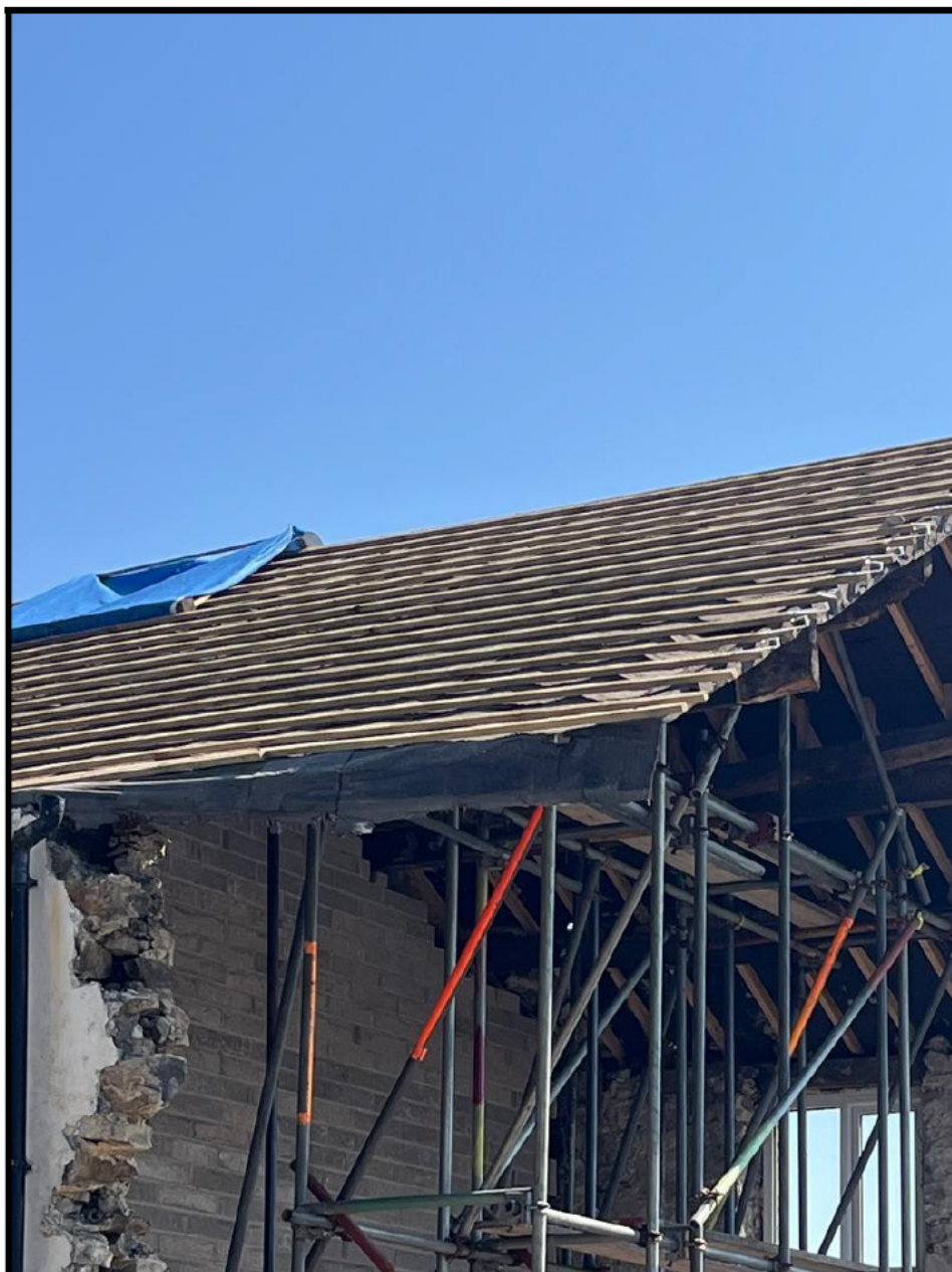
South gable wall removed.
