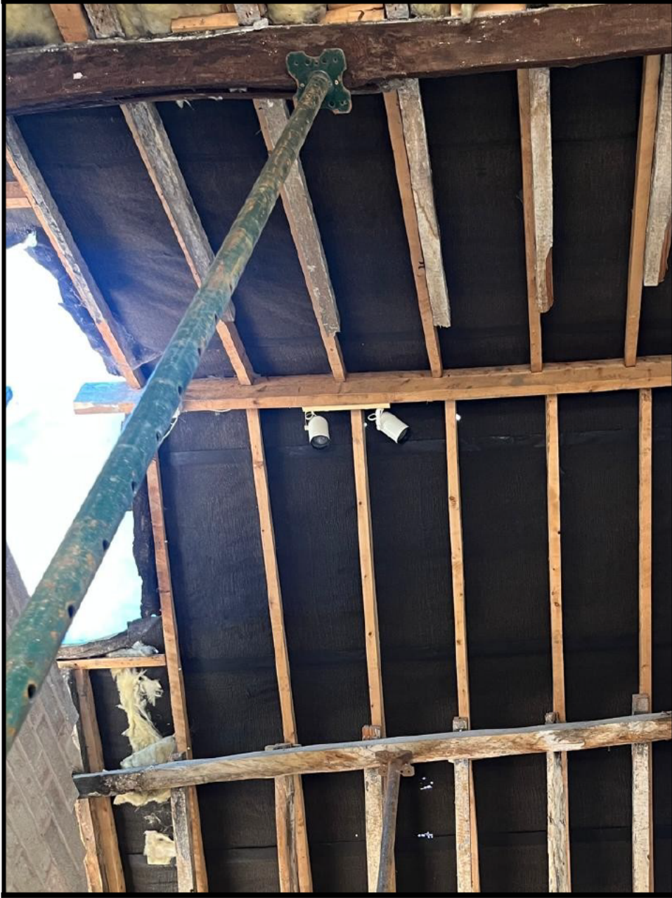
Decayed first floor removed and roof structure exposed.
