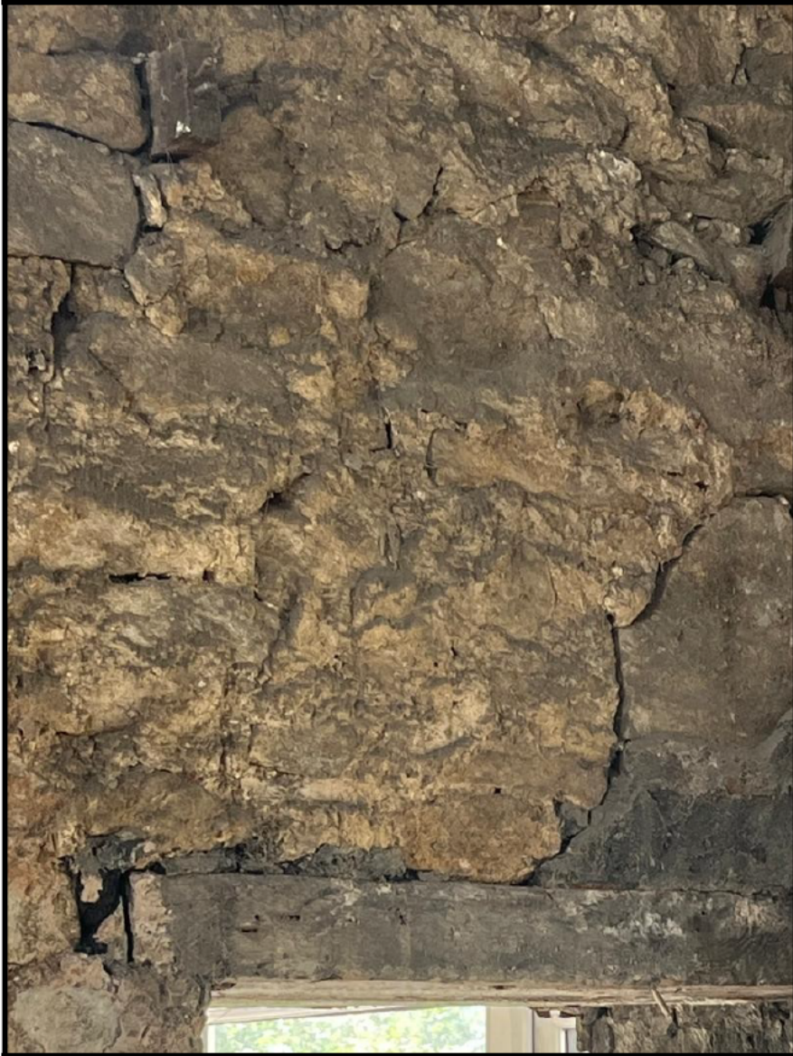
Doorway between living room and sun room
