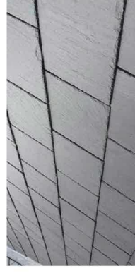
GRAY SLATE ROOFING
