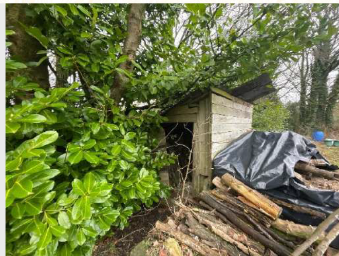
Photograph 18: Building 2; Freestanding wood store with negligible roosting potential.
