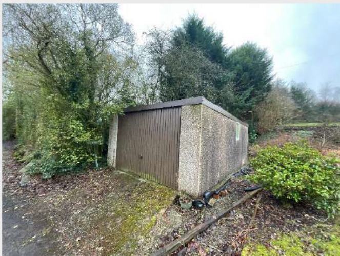
Photograph 19: Building 4; fixed garage with negligible roosting potential .
