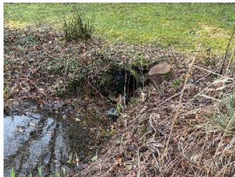
Figure 4 – Culverted watercourse feeding into the pond shown on figure 3.
