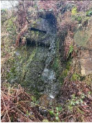
Figure 17 – Looking south shallow bedrock was noted in the cliff face beyond the southern site boundary.
