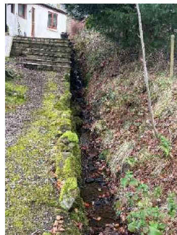
Figure 6 – Looking south east along the boundary showing the presence of a stream which was noted to become culverted and feed the pond.
