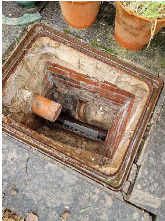
Figure 4 - Existing Surface water discharged to public sewer
