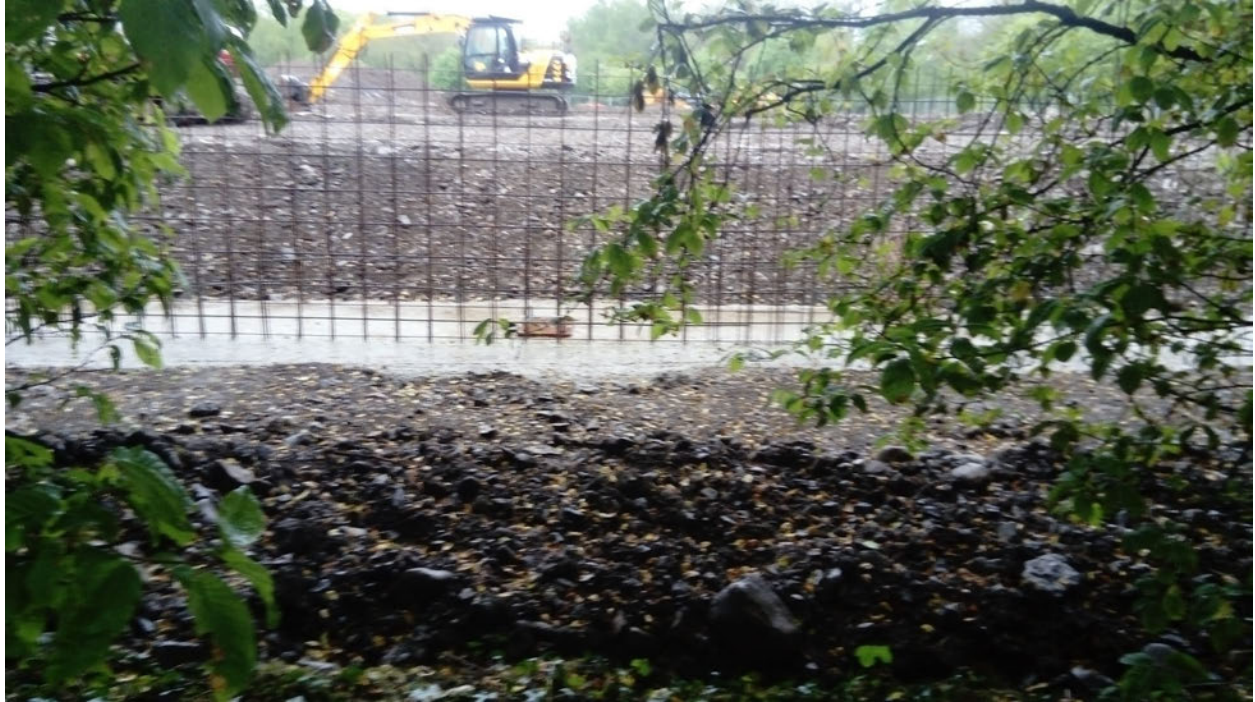
Figure 1 Twin Brook Business Park Land Raising during construction
