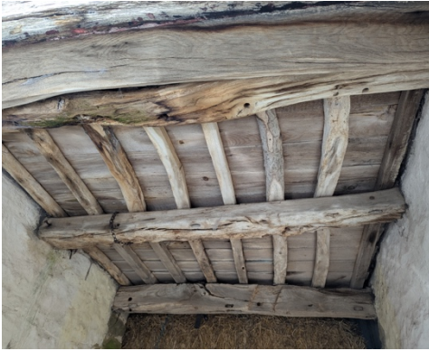
Figure 10: View of historic timbers
