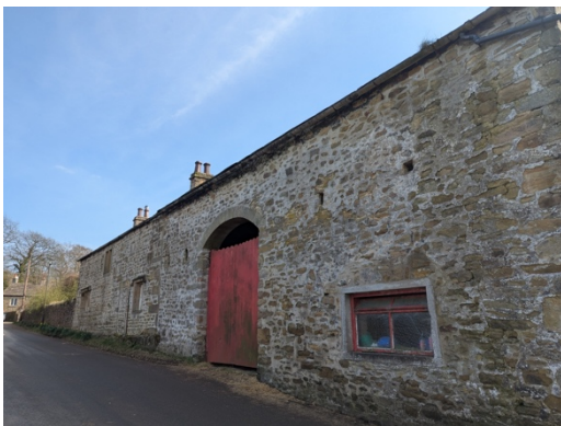
Figure 2: View of the principal elevation
