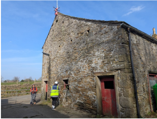
Figure 4: View of the west facing elevation
