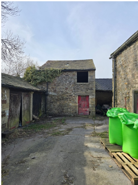
Figure 12: View of the rear yard
