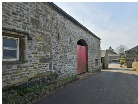
Figure 17: View looking west along the main road
