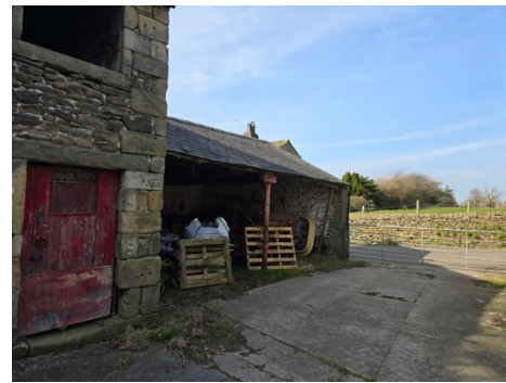
Figure 13: View of the rear yard
