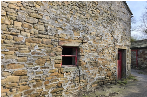
Figure 6: View of the west facing elevation
