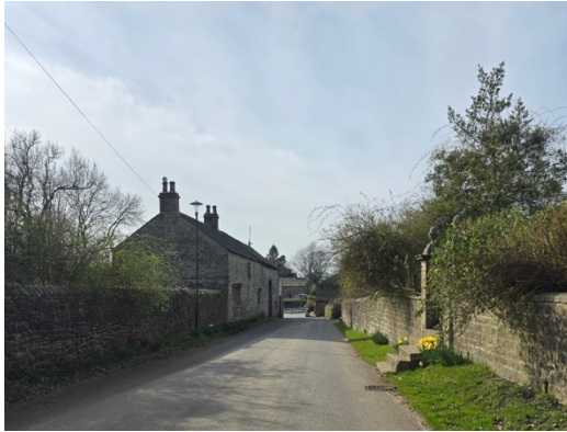
Figure 18: View looking west along the main road
