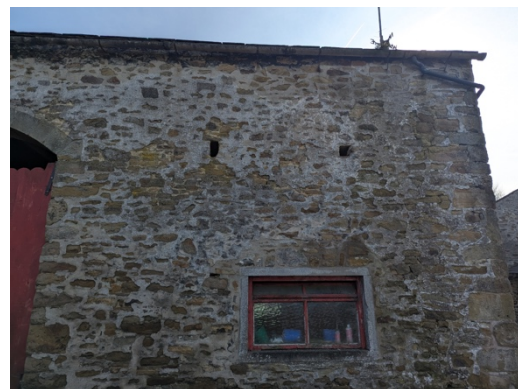
Figure 3: View of the principal elevation
