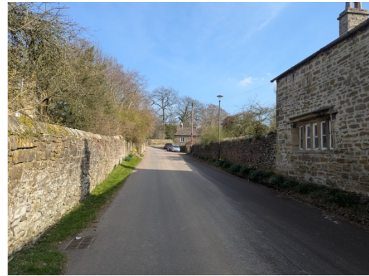
Figure 15: View looking west along the main road
