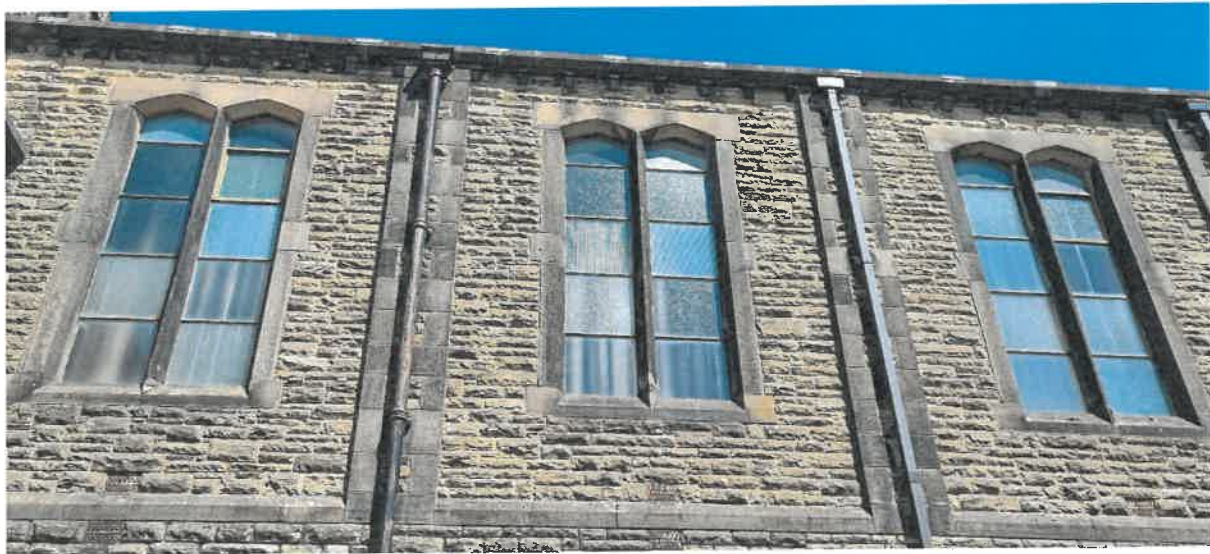
Windows 4, 5, 6 – South Elevation
