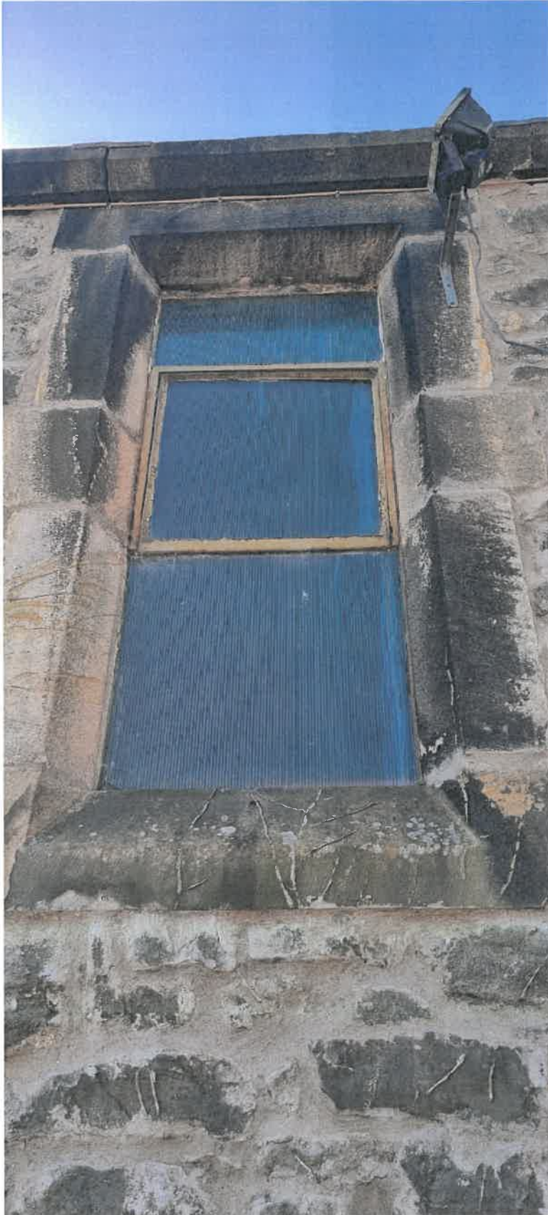
Window 7 - North Elevation
