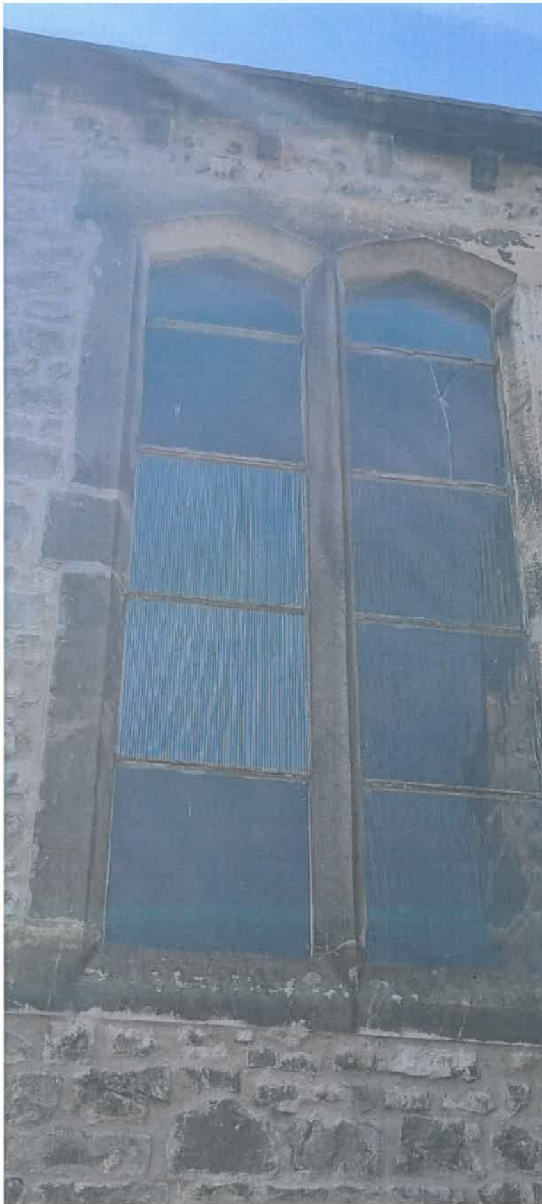
Window 1 - North Elevation
