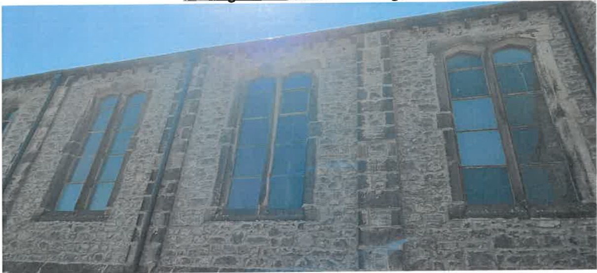
Windows 1, 2, 3 – North Elevation
