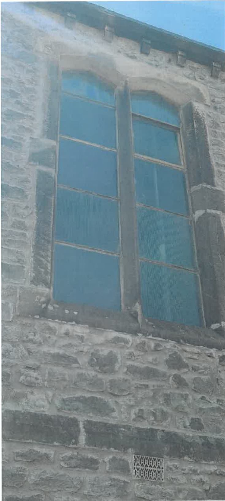
Window 2 - North Elevation
