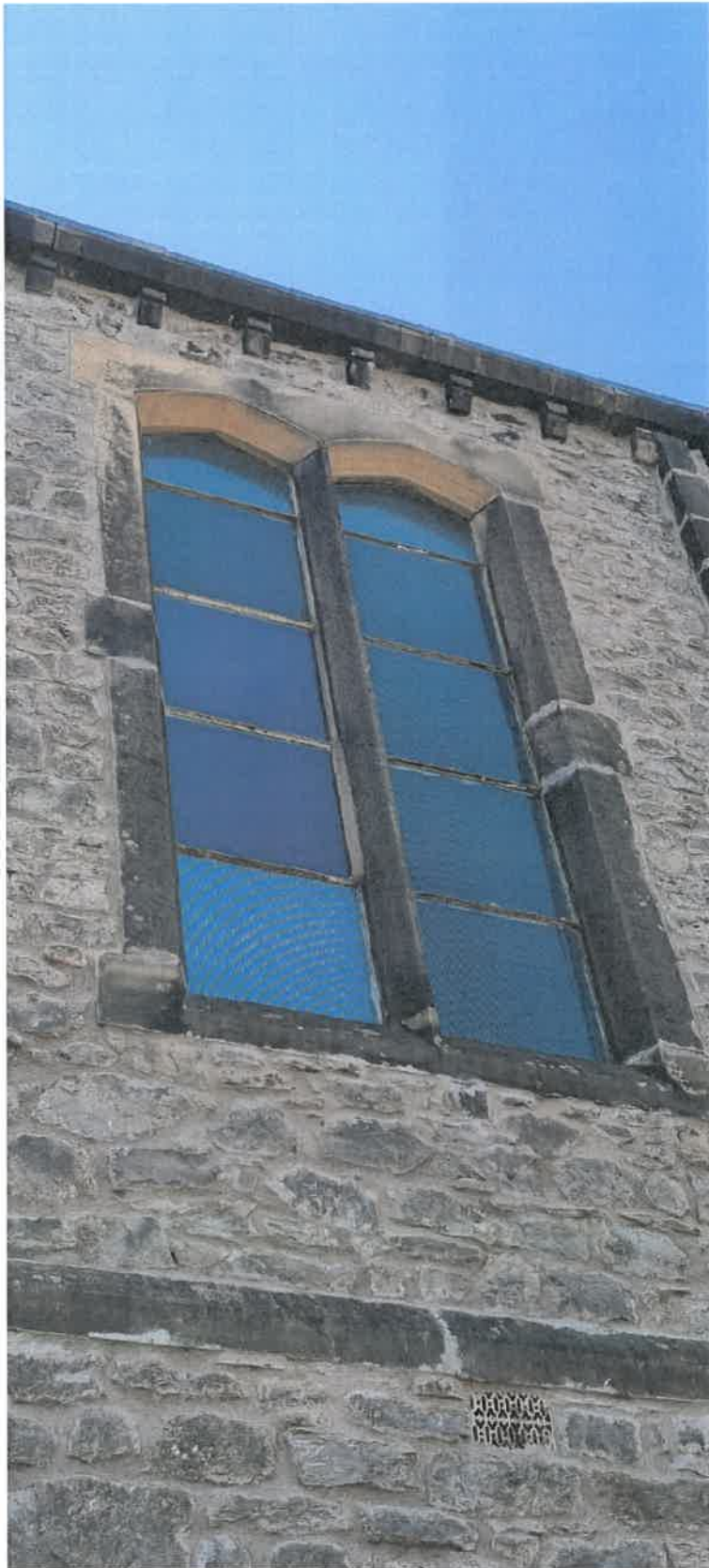
Window 3 - North Elevation
