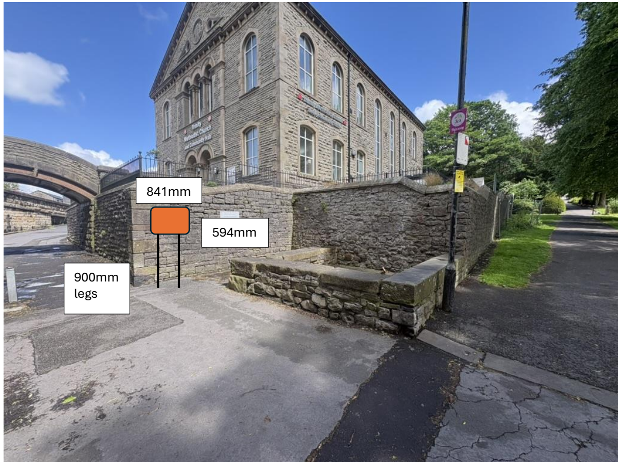
Photo showing the proposed location of the Information Board
