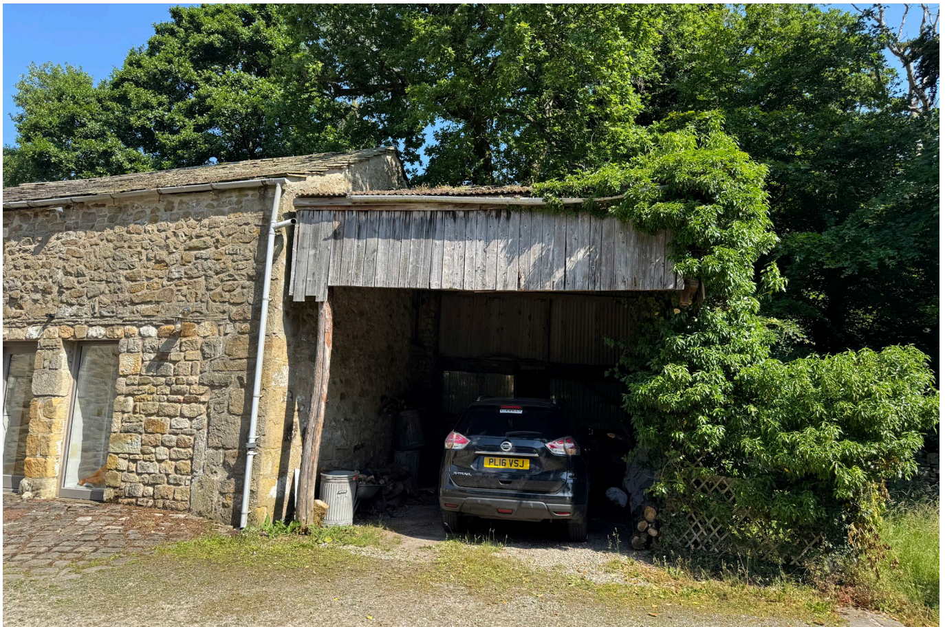
Figure 5. Derelict cart shed
