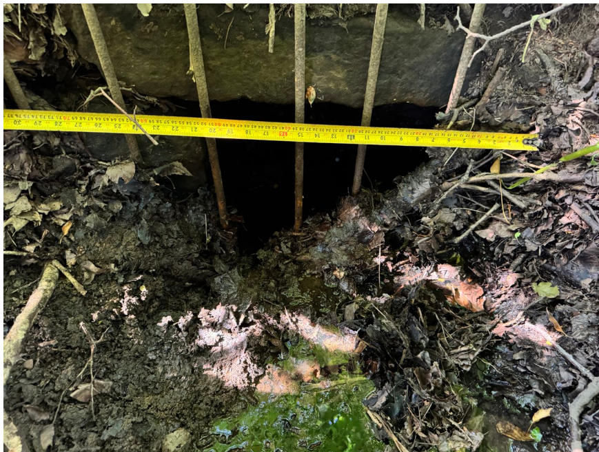
Fig 4 Width of culvert
