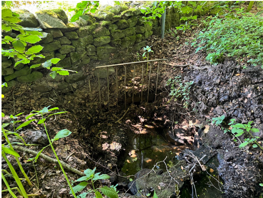
Fig 3 North end of culvert
