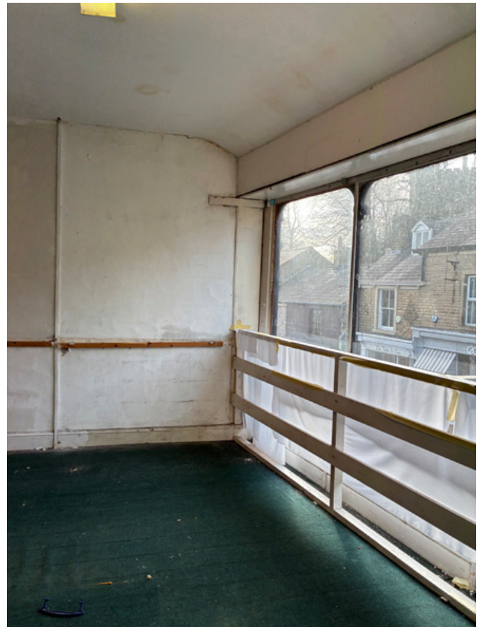
Existing First Floor Of Building (Fig 3)
