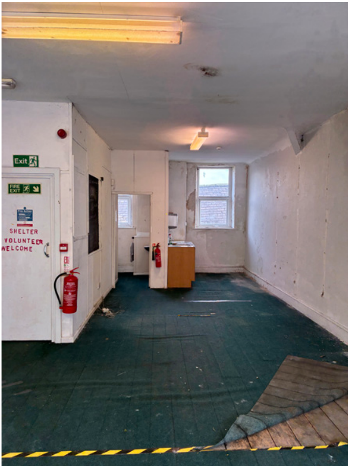
Existing First Floor Of Building (Fig 3)
