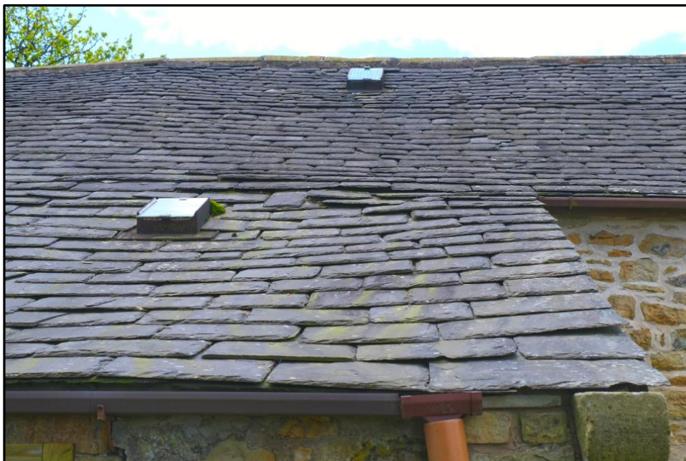
Image 2. Roof coverings on barn building (north elevation).
