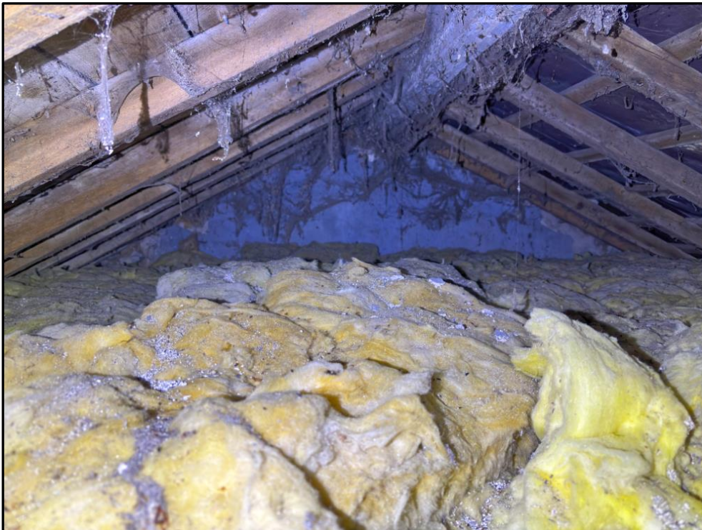
Image 4. Roof void of dwelling house, no connection to adjoining barn building.
