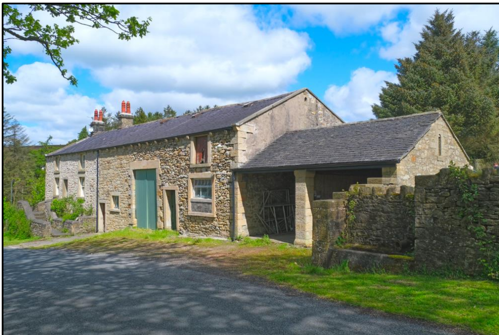
Image 1. South elevation of Cowley Brook Farm showing dwelling house (lhs), barn (middle) and car ports(rhs).
