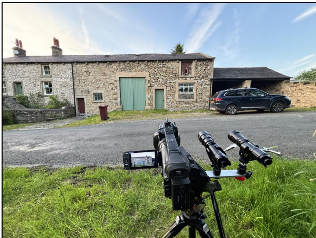
Image 10. View of south elevation prior to bat emergence survey.
