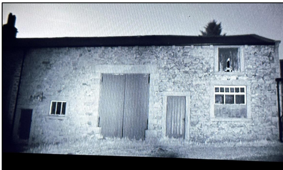
Image 11. View of south elevation at end of bat emergence survey.
