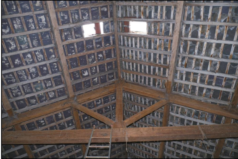
Image 3. Roof underside of barn, unlined with roof lights (limited sheltered dark spaces)
