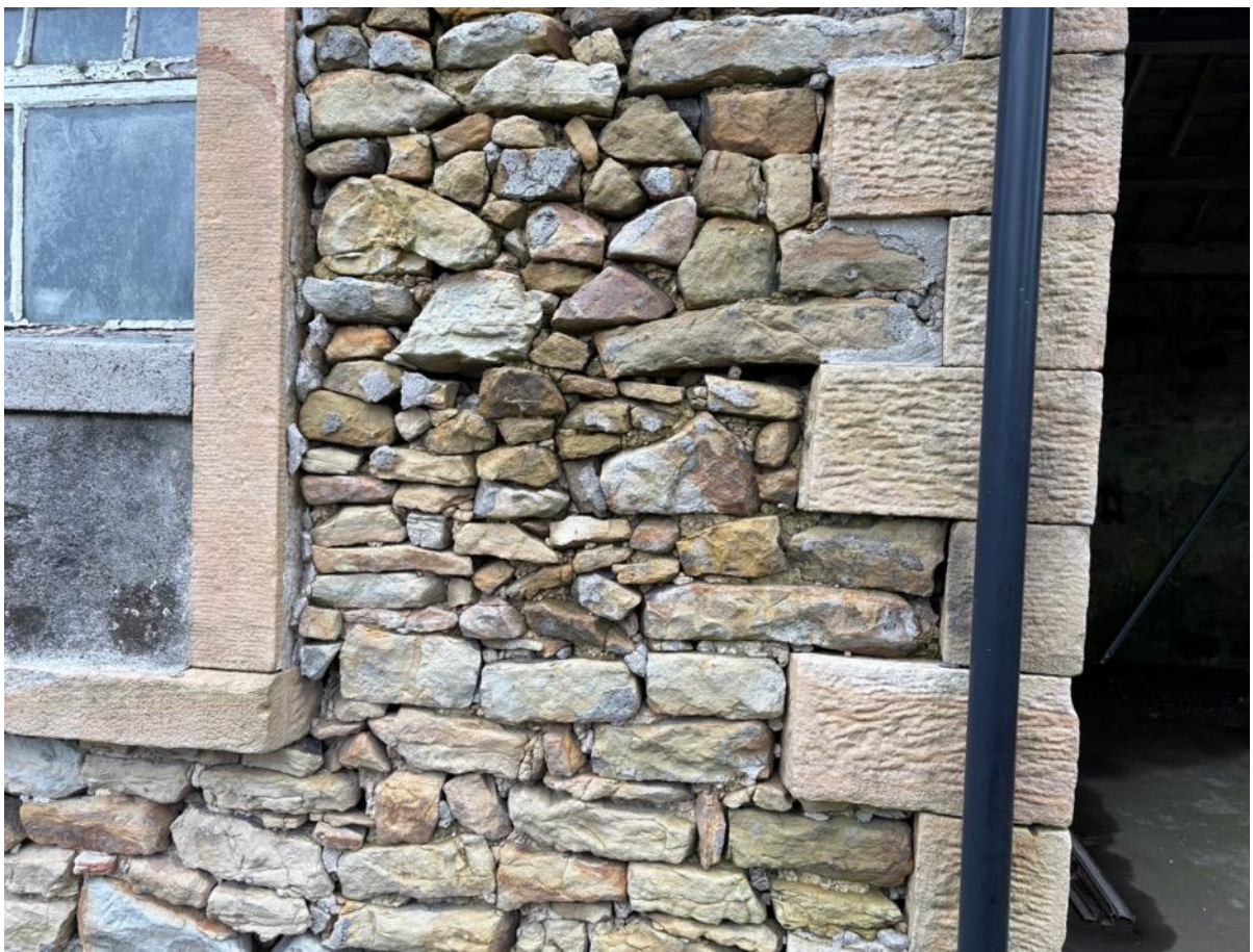
Photo 11 – Stonework to South West Elevation
