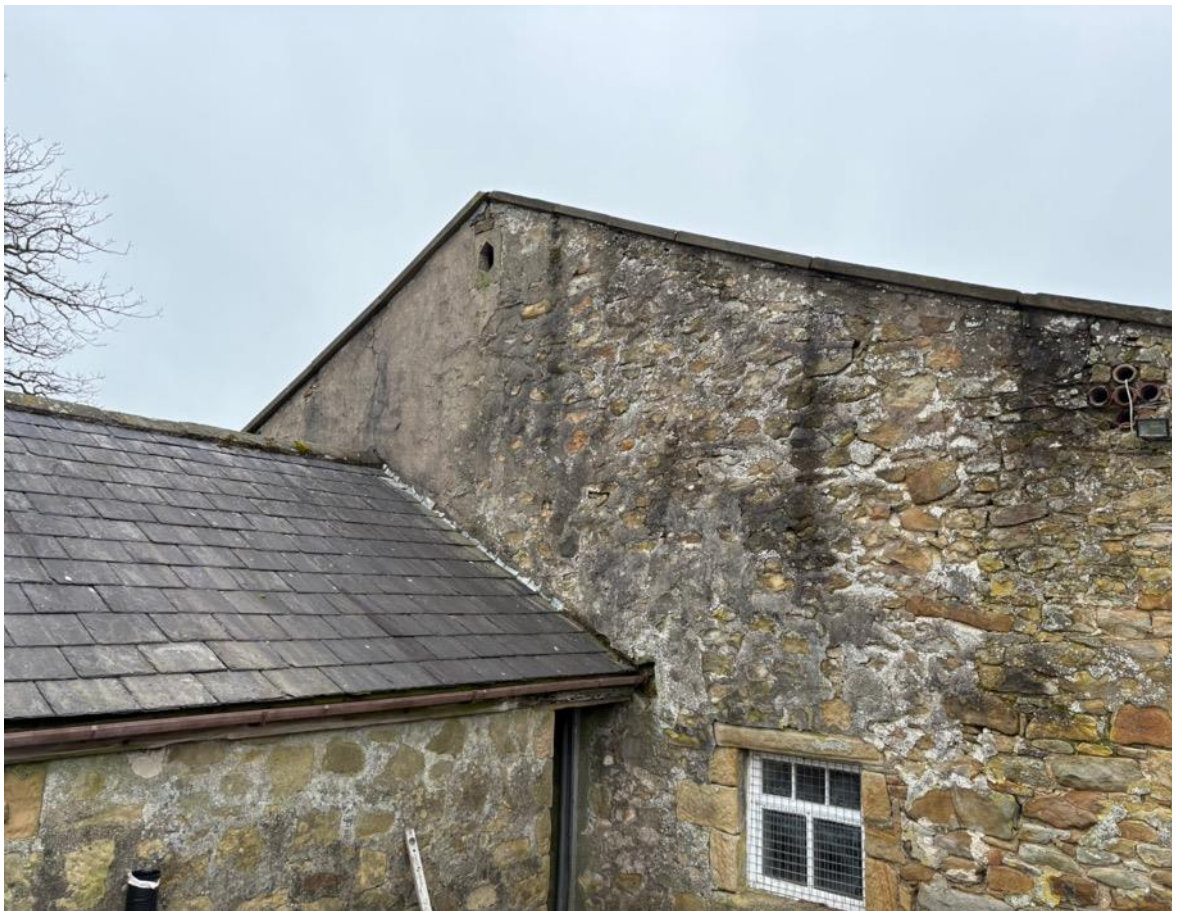
Photo 20 – South East Gable
