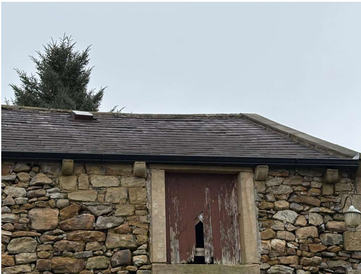
Photo 2 – South West Elevation and Roof
