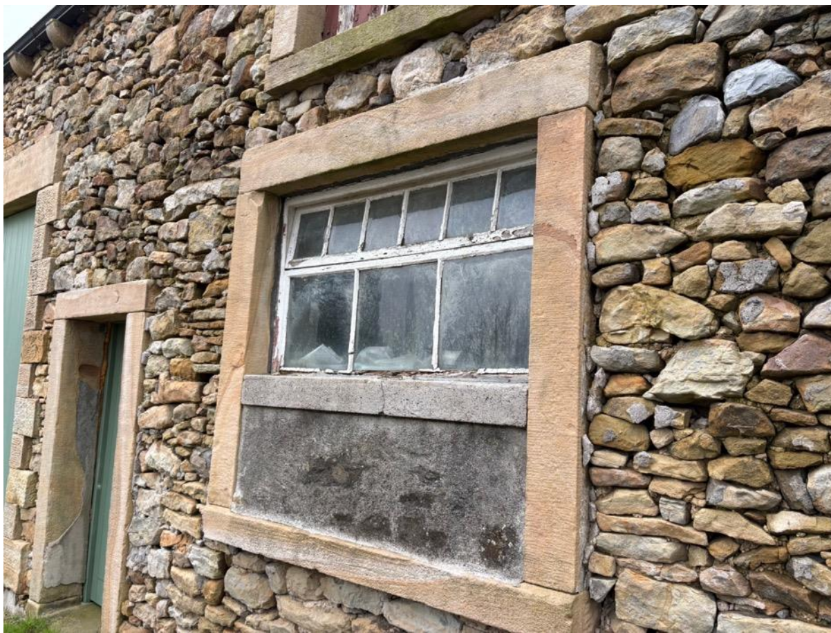
Photo 13 - Stonework to South West Elevation
