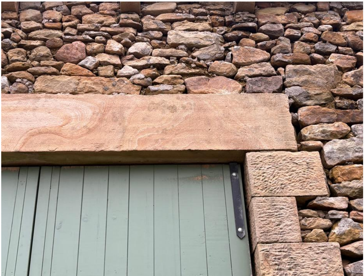
Photo 18 – Stone Lintel to main door to South West Elevation
