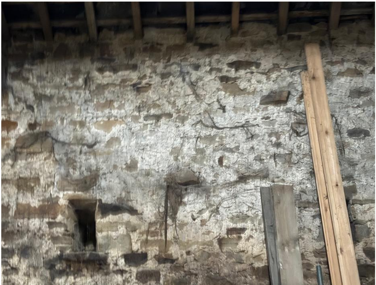
Photo 31 - Internal main barn
