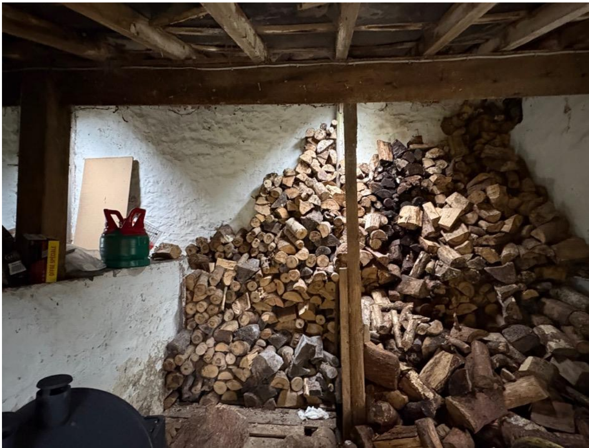
Photo 27 – Internal rear single storey
