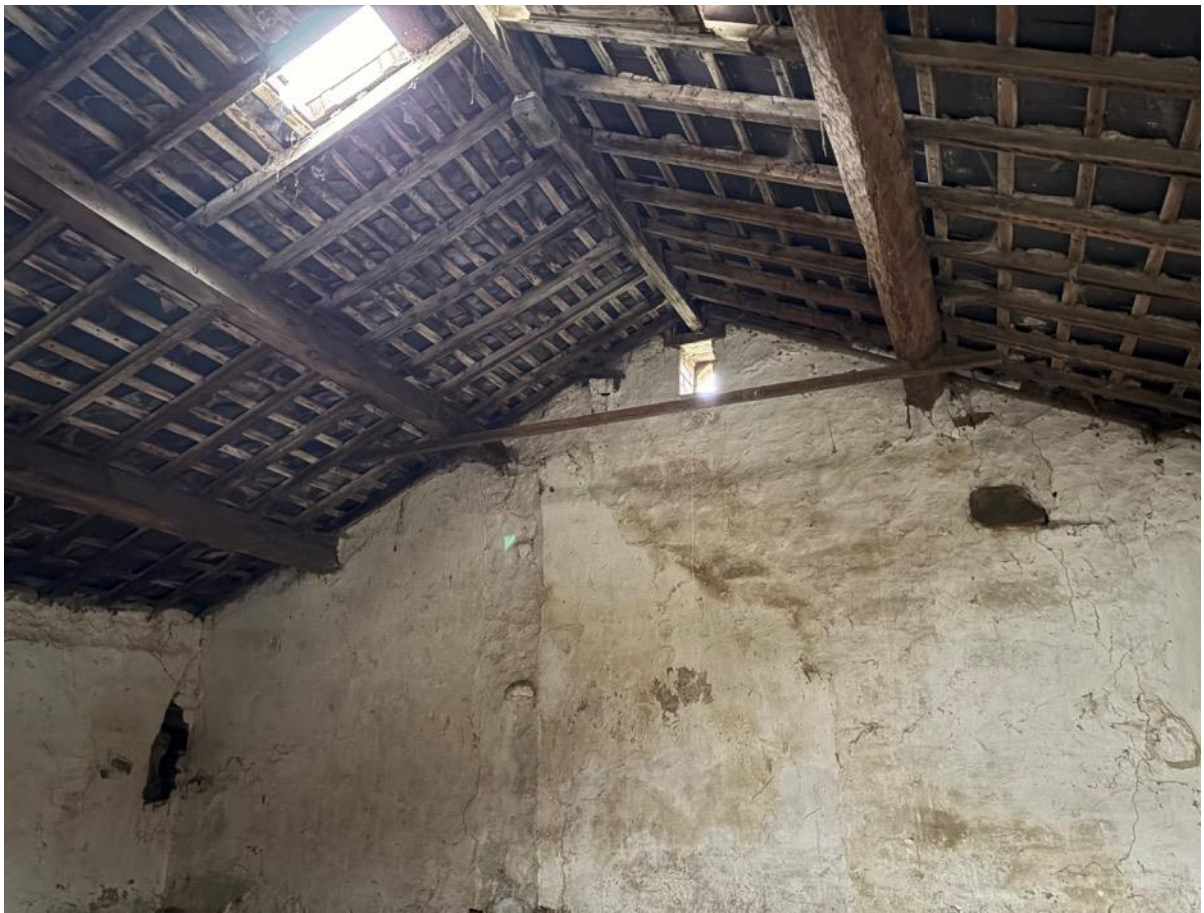
Photo 35 – Internal main barn roof
