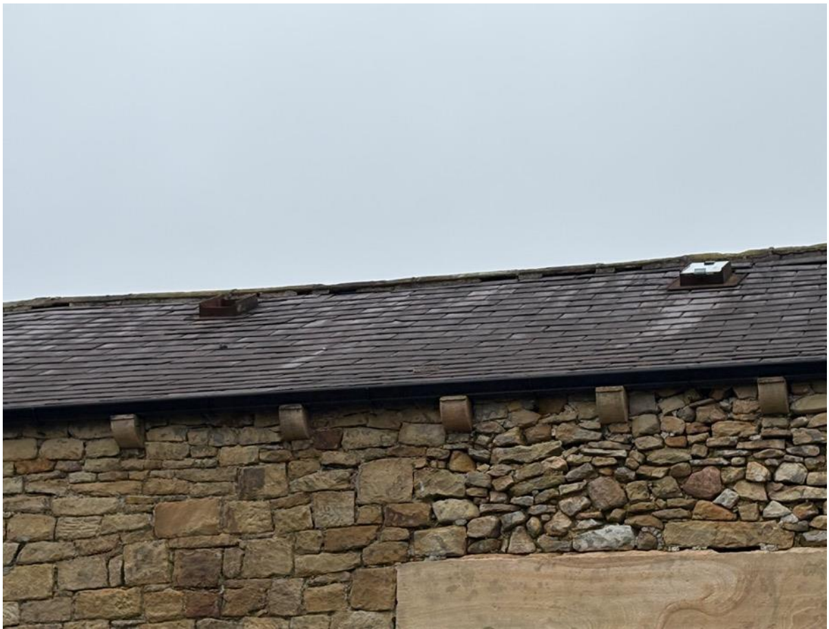
Photo 3- South West Elevation and Roof
