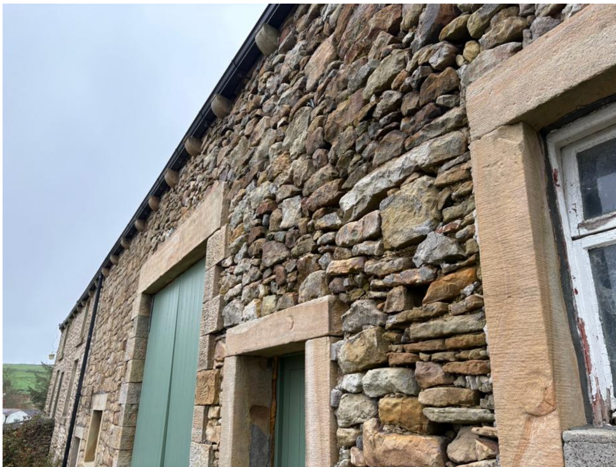
Photo 14 - Stonework to South West Elevation
