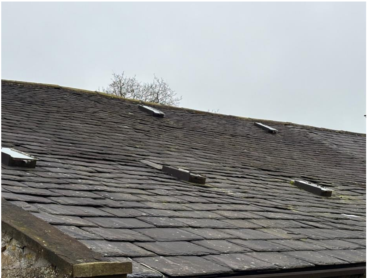
Photo 23 – Roof to North East Elevation
