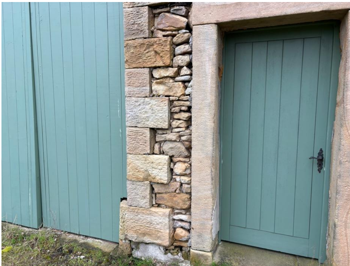
Photo 15 - Stonework to South West Elevation
