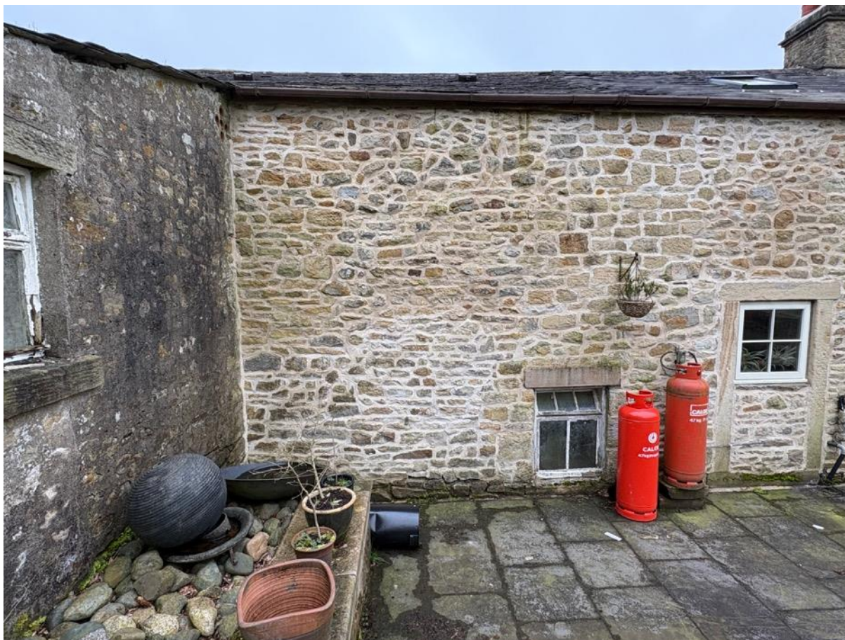
Photo 26 – North East Elevation adjacent to farmhouse
