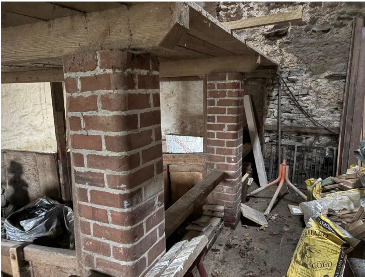
Photo 39 – Mezzanine with brick pillars in main barn
