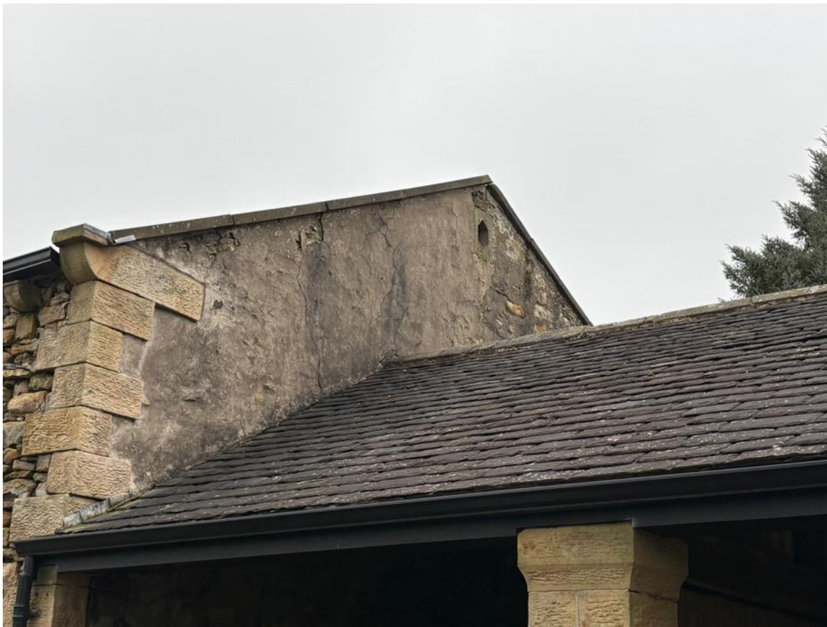
Photo 6 – South East Gable and Roof to Open Garage/Storage at South East End
