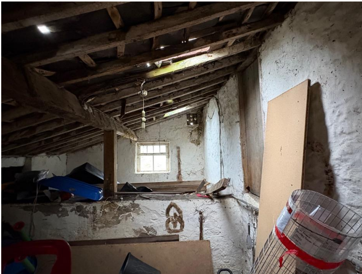
Photo 28 - Internal rear single storey
