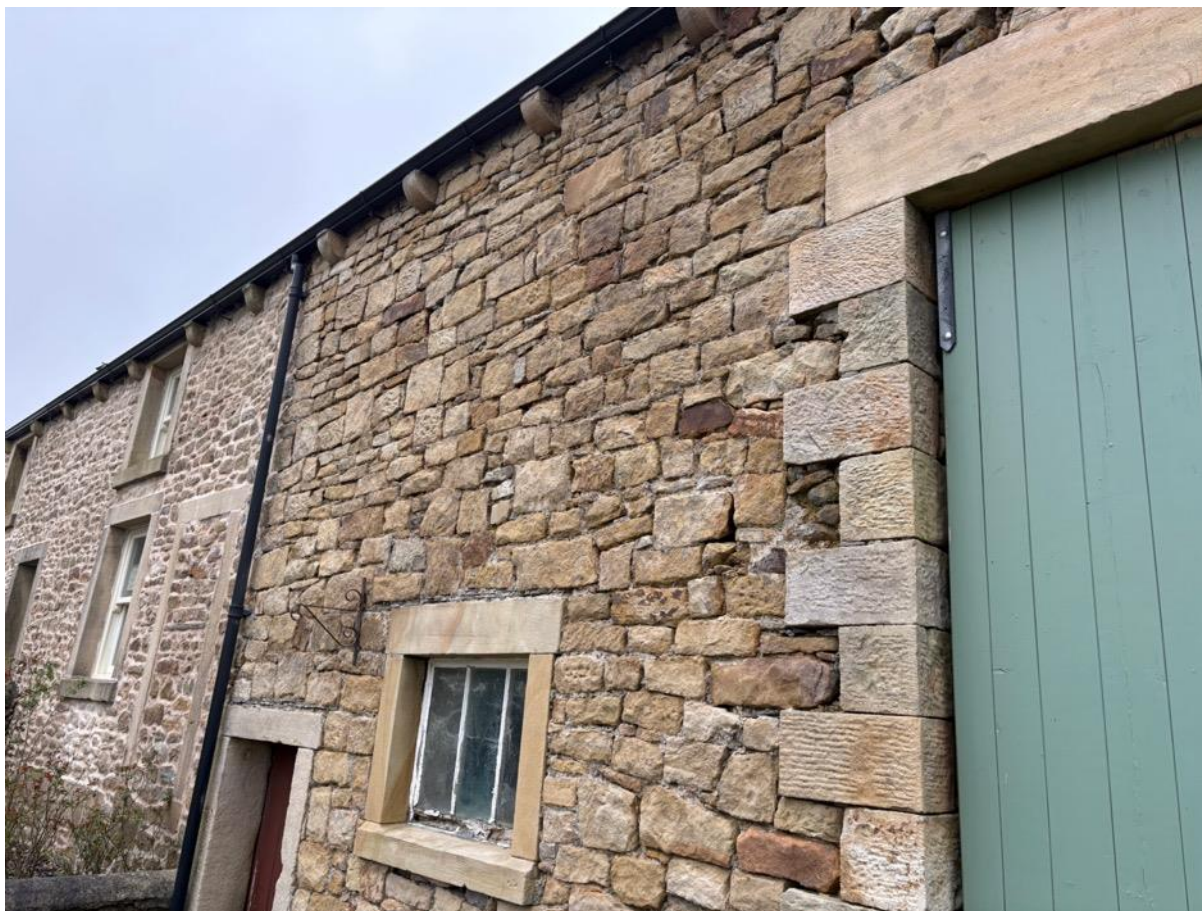
Photo 16 - Stonework to South West Elevation
