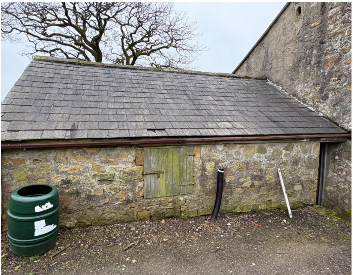
Photo 19 – North East Elevation to garage/storage
