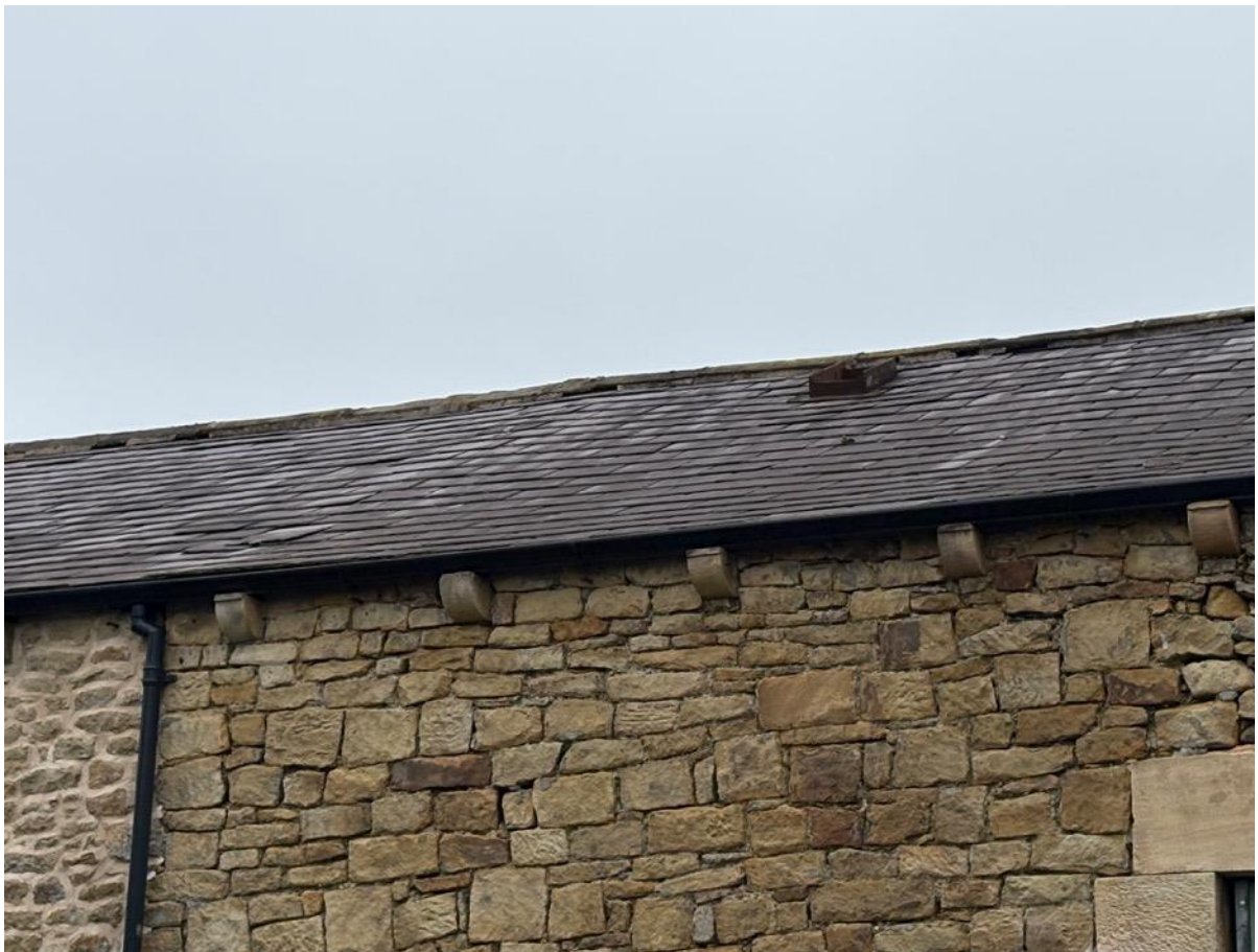
Photo 4 - South West Elevation and Roof
