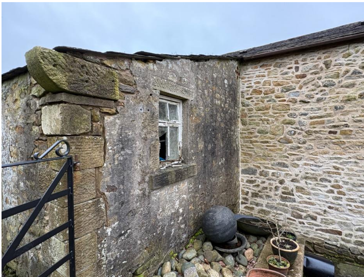
Photo 25 – North West Elevation or rear single storey section
