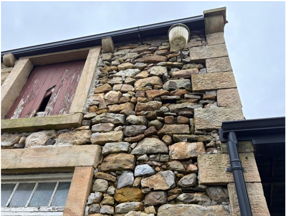
Photo 12 - Stonework to South West Elevation
