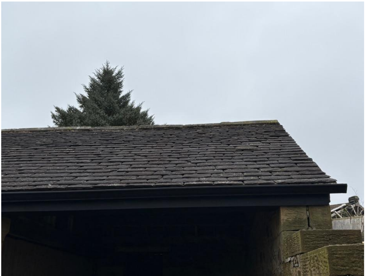
Photo 7 – Roof to Open Garage/Storage at South East End
