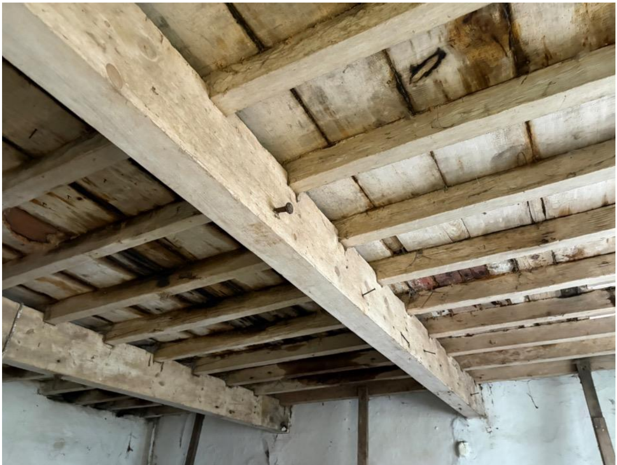
Photo 30 – Internal main barn
