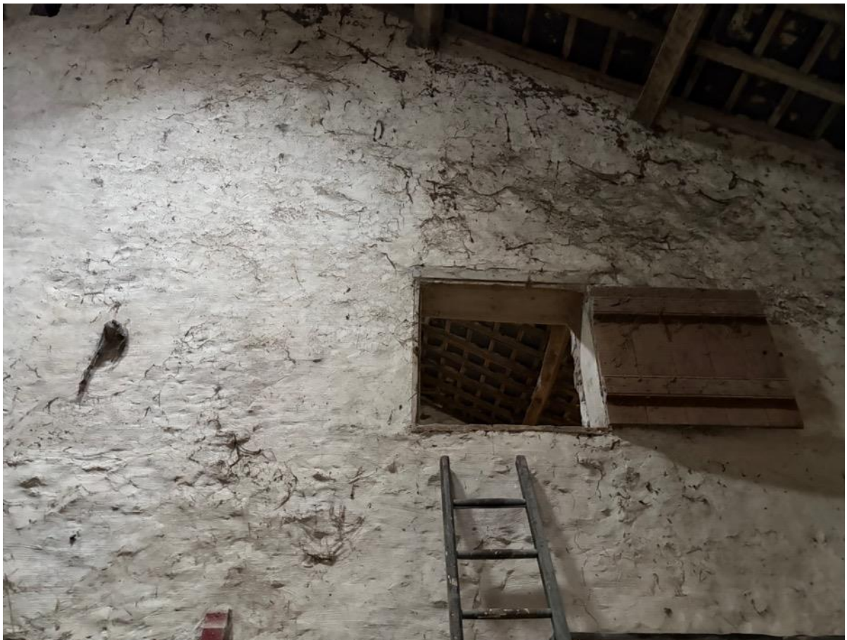
Photo 36 - Internal main barn – Dividing wall main barn
