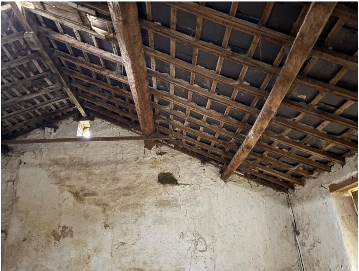
Photo 34 - Internal main barn roof
