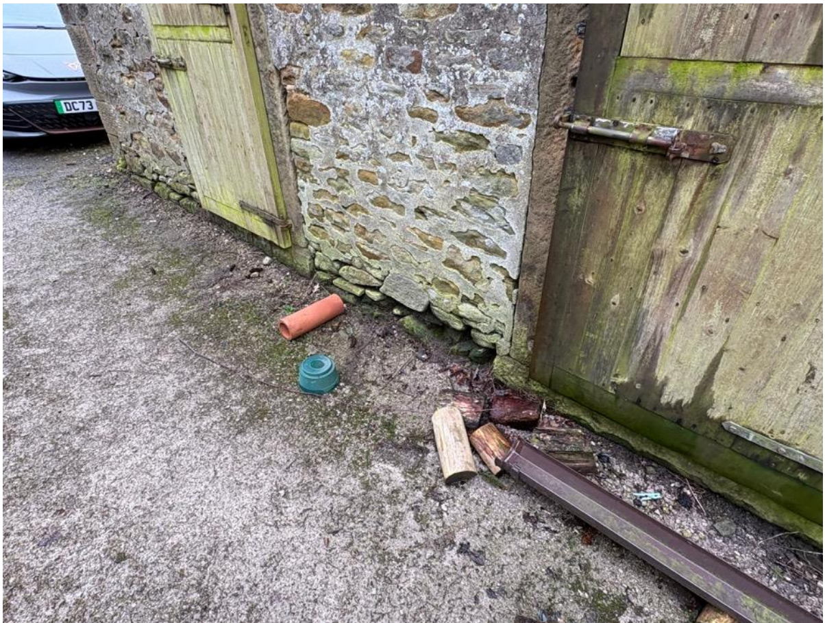
Photo 24 – North East Elevation
