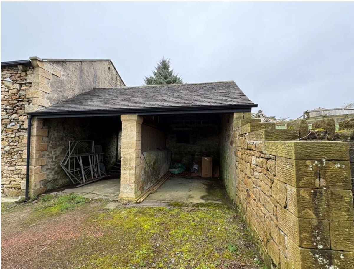
Photo 5 – South West Elevation – Open Garage/Storage at South East End
