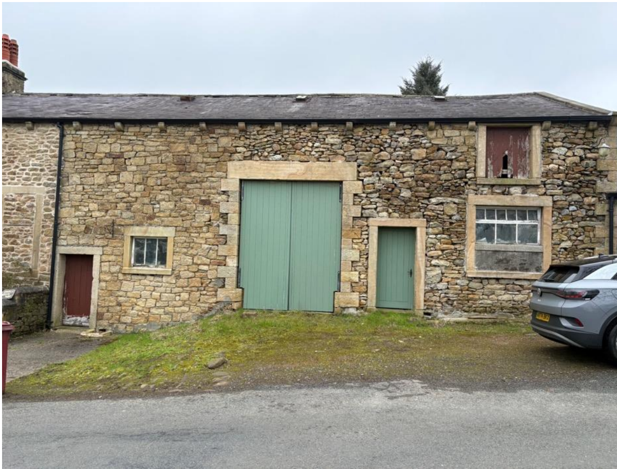
Photo 1 - South West Elevation
