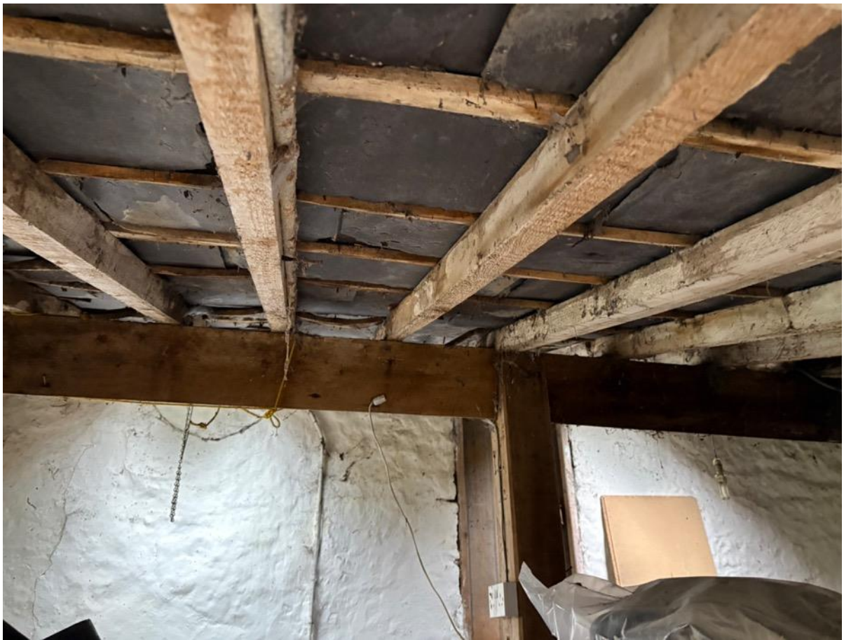
Photo 29 - Internal rear single storey
