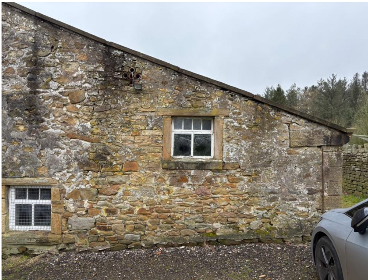
Photo 21 – South East Gable
