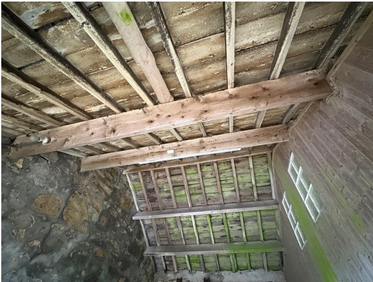
Photo 10 – internal of Roof to Open Garage/Storage at South East End
