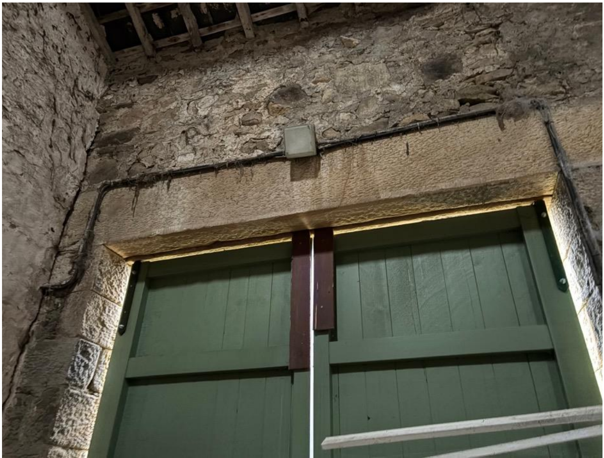
Photo 41 – Main door internal
