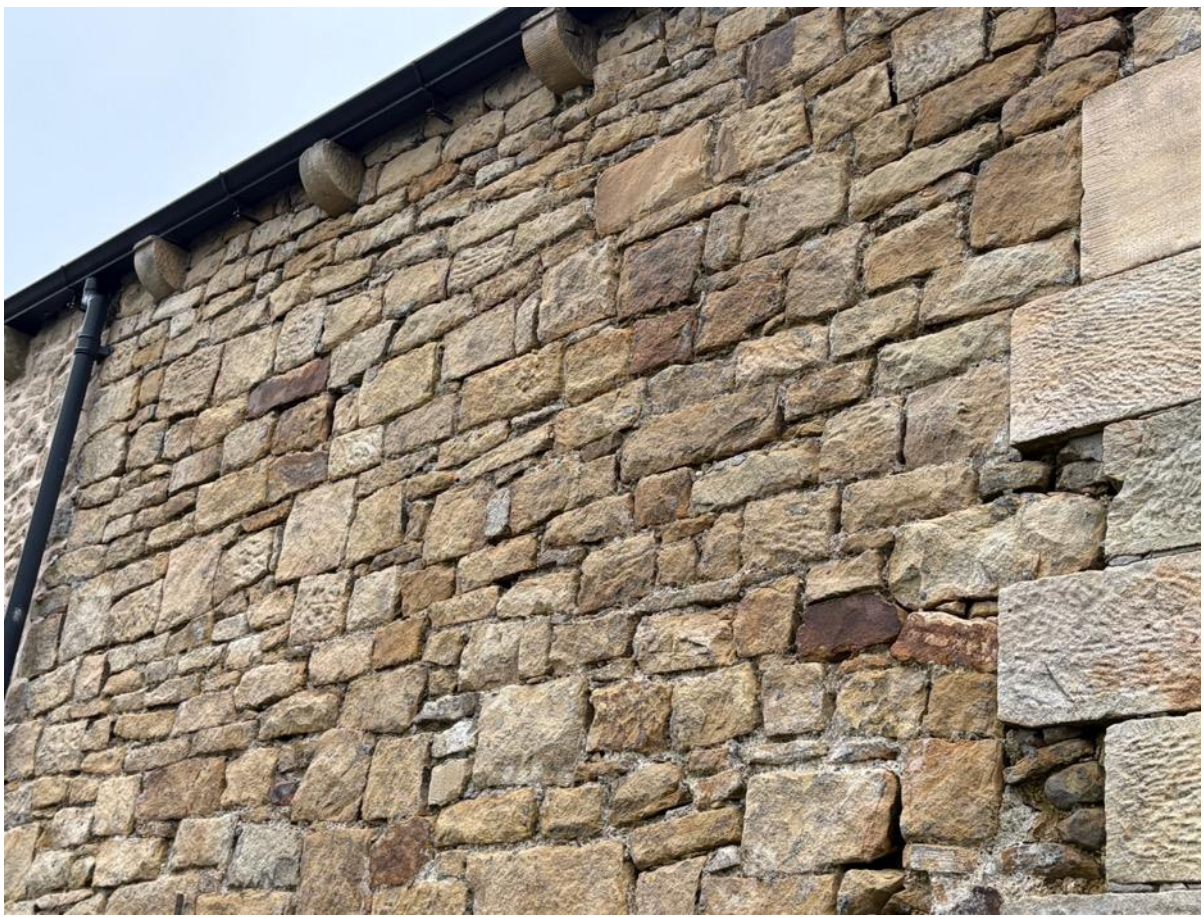
Photo 17 - Stonework to South West Elevation
