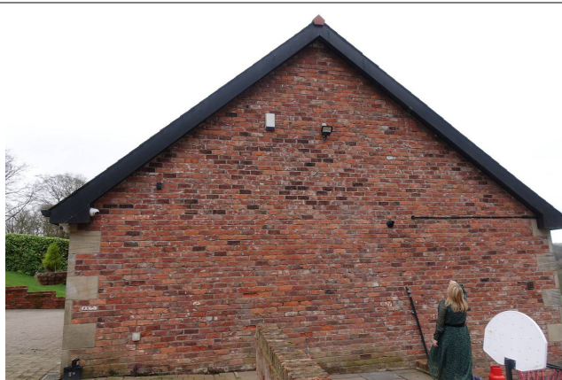
Western gable end
