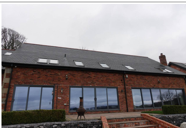
South facing facade
