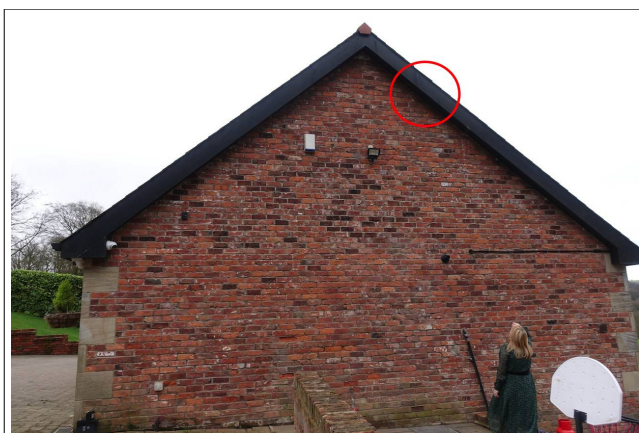
Location of roost entrance on western gable
