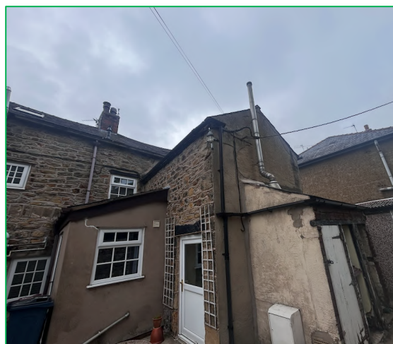
The southwest elevation of the building
