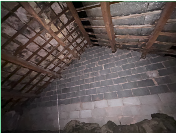
The large loft void; the roof is unlined on the northeast elevation.
