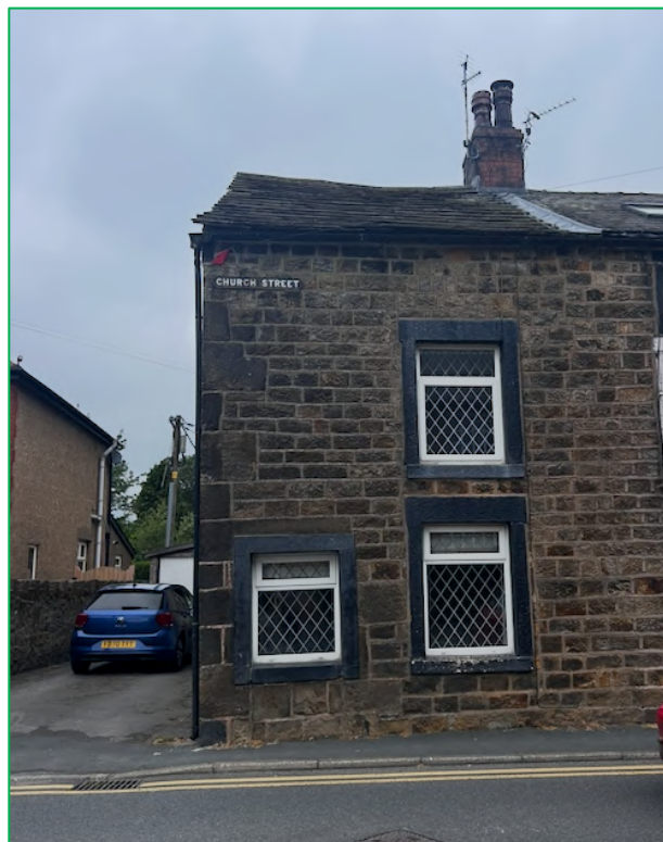
The northwest elevation of the building
