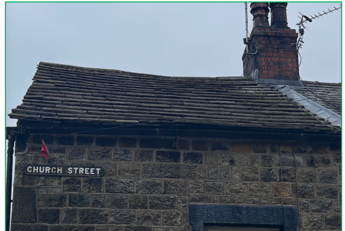
The roof on the northeast elevation
