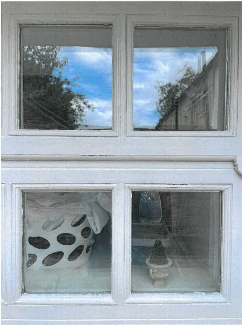
Photographs to illustrate the appearance of the windows, showing outside and inside views.
