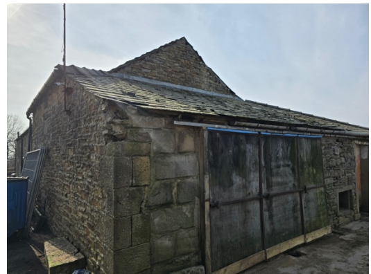
Figure 7: View of the east facing elevation
