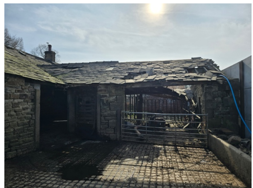
Figure 9: View of the east facing elevation
