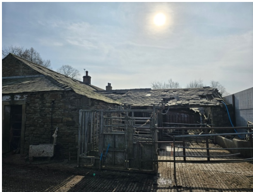
Figure 6: View of the east facing elevation
