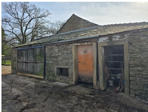
Figure 8: View of the east facing elevation
