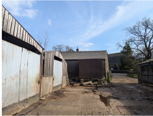
Figure 10: View of the rear yard
