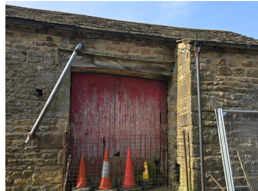
Figure 5: View of the cart shed entrance
