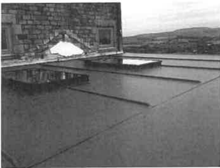
Photo 1c – Flat roof roofing
